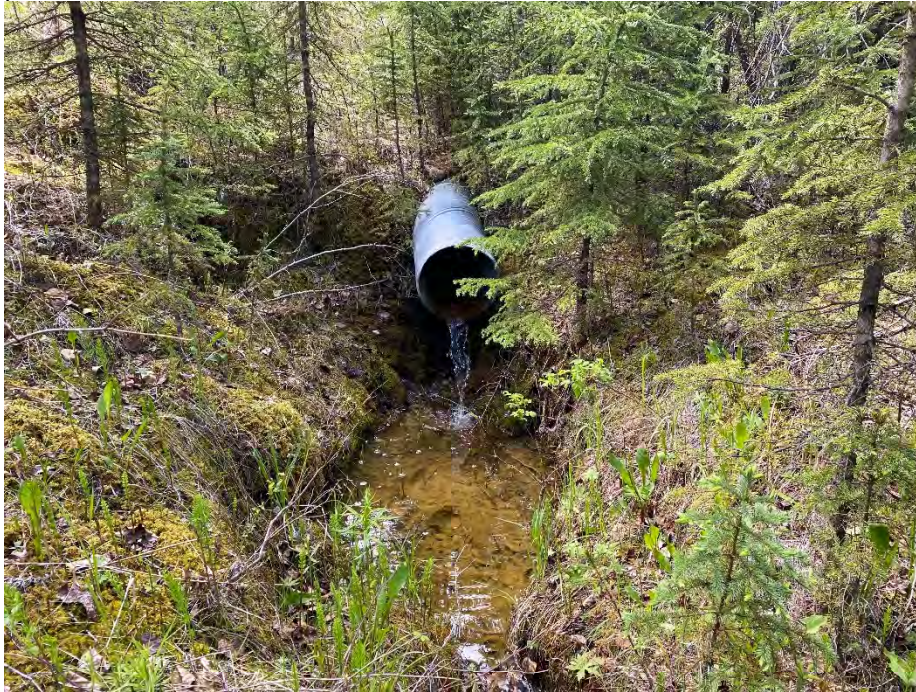
Photo 6: Water flowing under 780 mm diameter culvert. Looking southeast.
