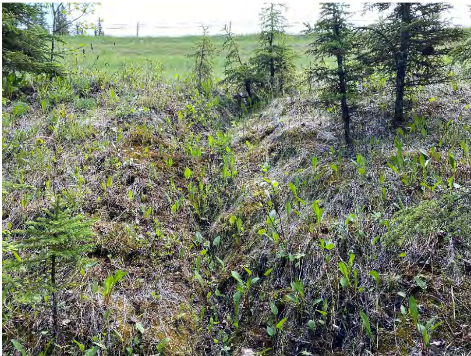
Photo 7: Vegetated erosion gully on southwest side of highway. Looking east.
