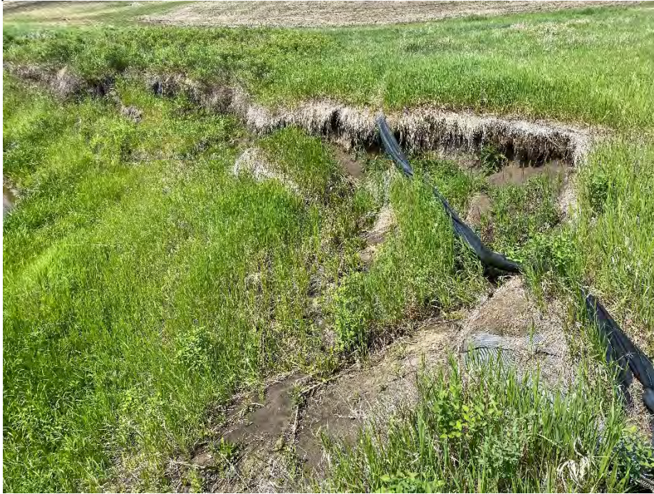
Photo 9: Slumping of slopes at the northwest bend in the river. Looking northwest.
