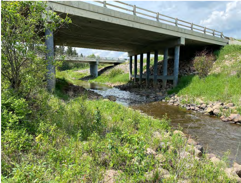
Photo 1: Highway 43 bridges and river embankments. Looking west.
