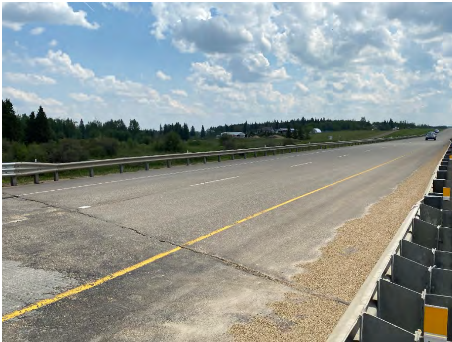
Photo 4: Pavement surface of the westbound bridge on Highway 43. Looking northwest.
