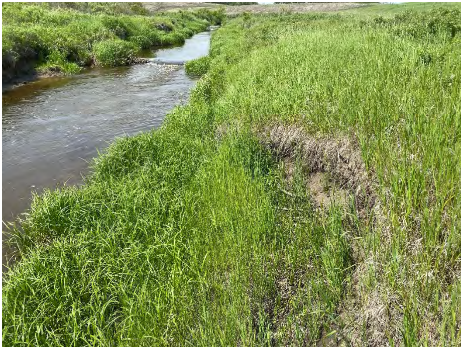
Photo 8: Slumping of crack noticed during last inspection south from SI14-27. Looking northwest.
