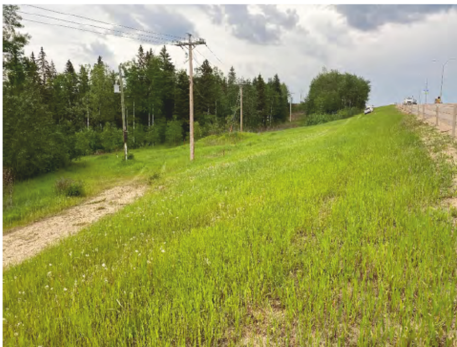
Photo 6: Overall view of north slope near highway. Looking southeast.
