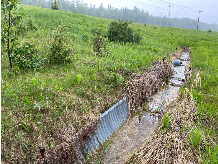
Photo 7: Half-culvert on north slope. Looking west.
