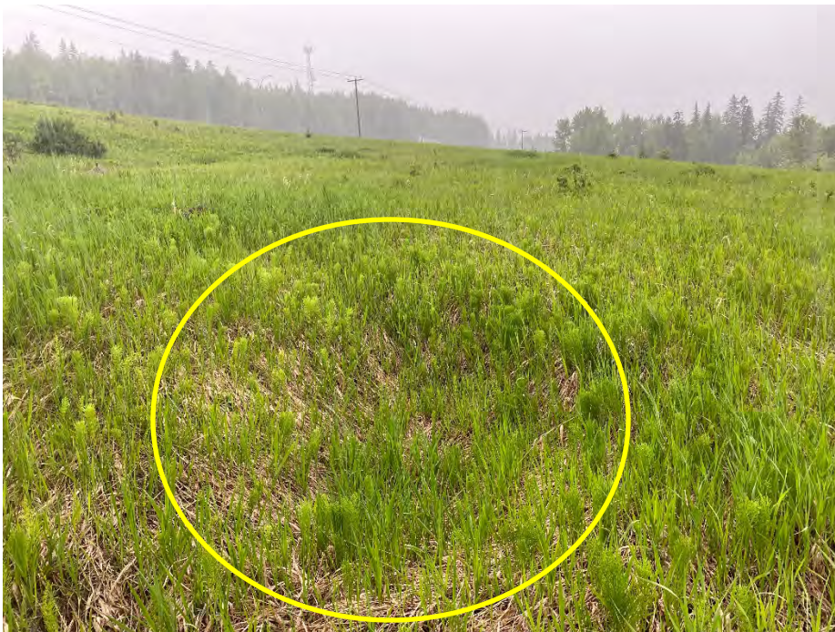
Photo 8: Depression in north slope between SI-12 and SP06-1. Looking west.
