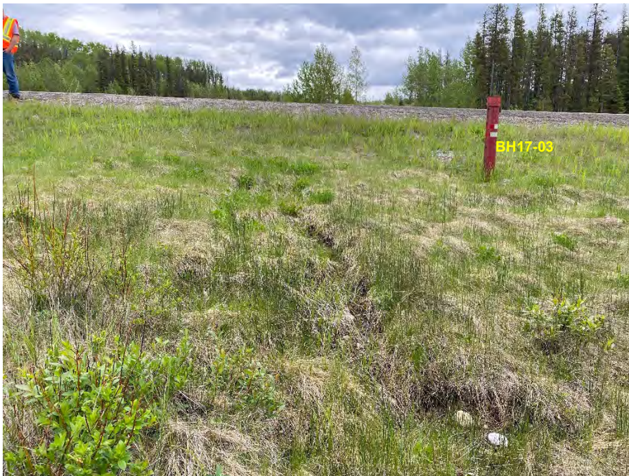
Photo 6: Seepage in vehicle track. 300 mm deep track. Looking northeast.
