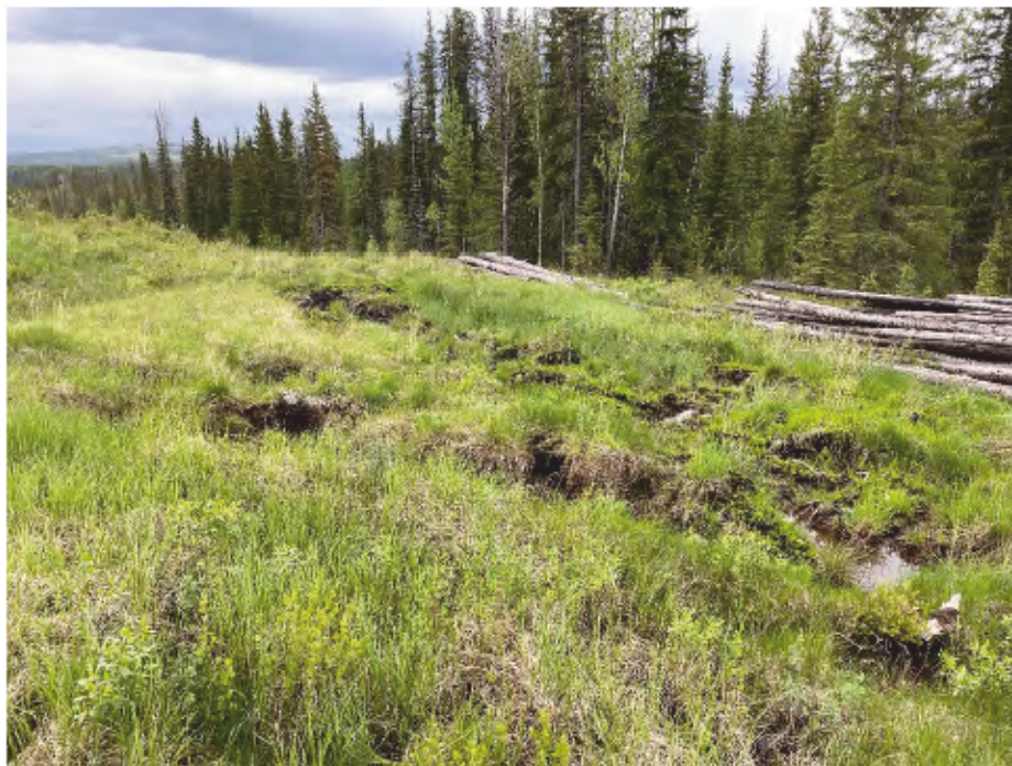
Photo 8: Erosion and ponded water in tree clearing area. Looking southeast.
