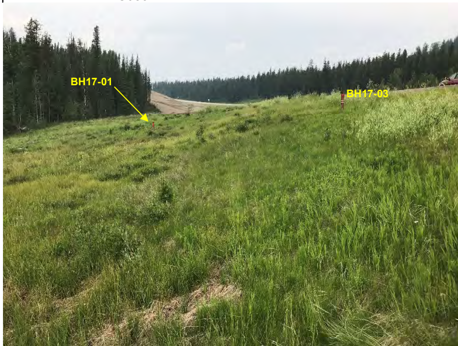
Photo 7: Overall view of south slope. Looking northwest.
