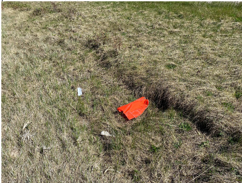
Photo 7: Possible sinkhole in the north ditch. Looking southeast.
