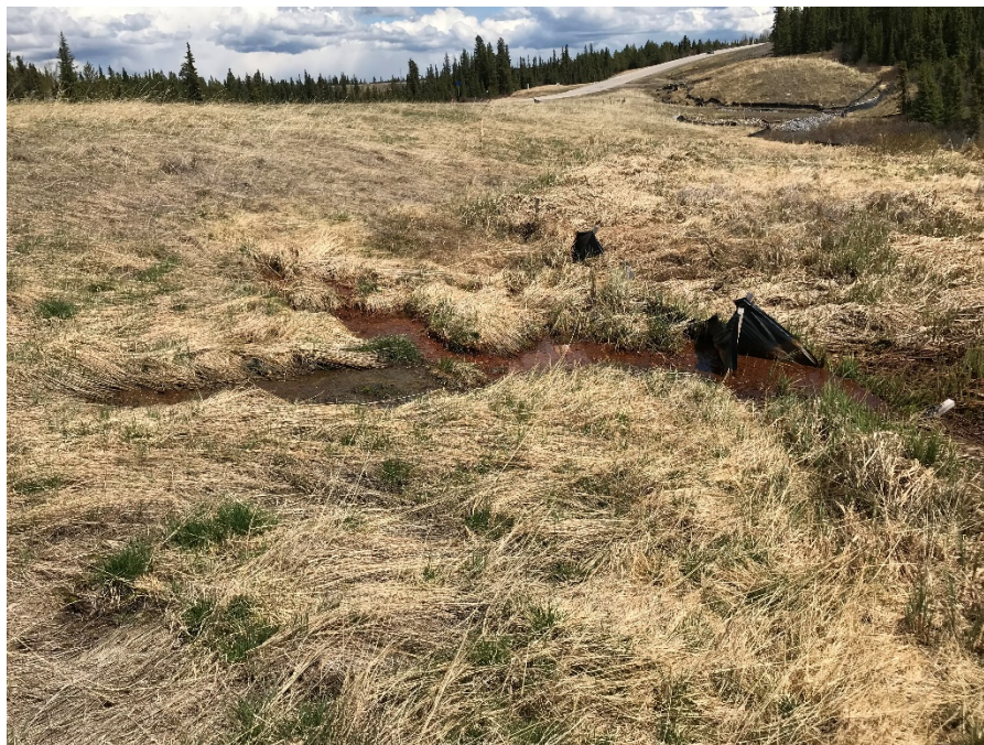
Photo 8: Seepage south of PZ7 near toe. Looking east.
