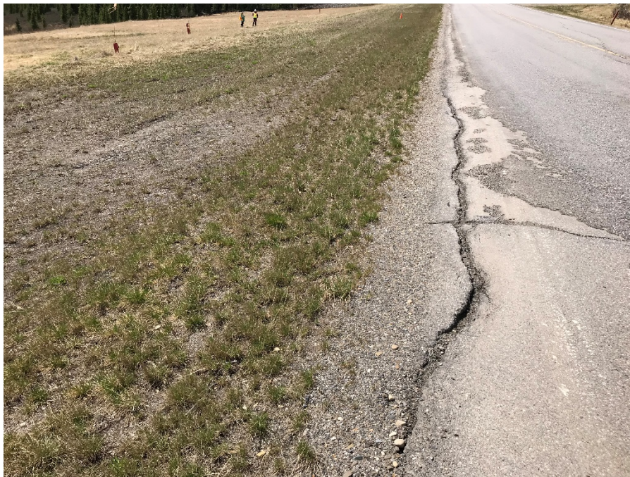
Photo 5: Pavement crack along shoulder at east end of patch. Looking west.
