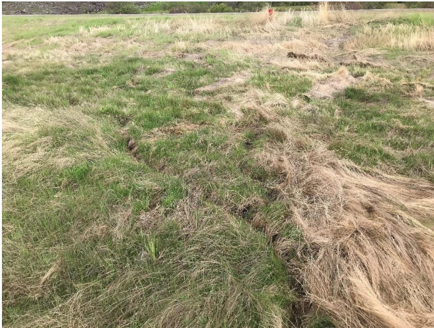
Photo 5: Erosion gully approximately 150 mm wide south of PZ7. Looking northwest.
