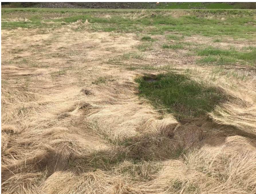
Photo 4: New seepage south of PZ6. Looking north.
