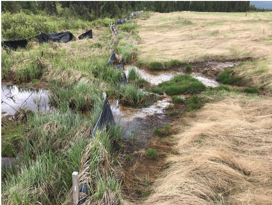
Photo 3: Flowing seepage along east end of silt fencing in repair area. Looking southwest.
