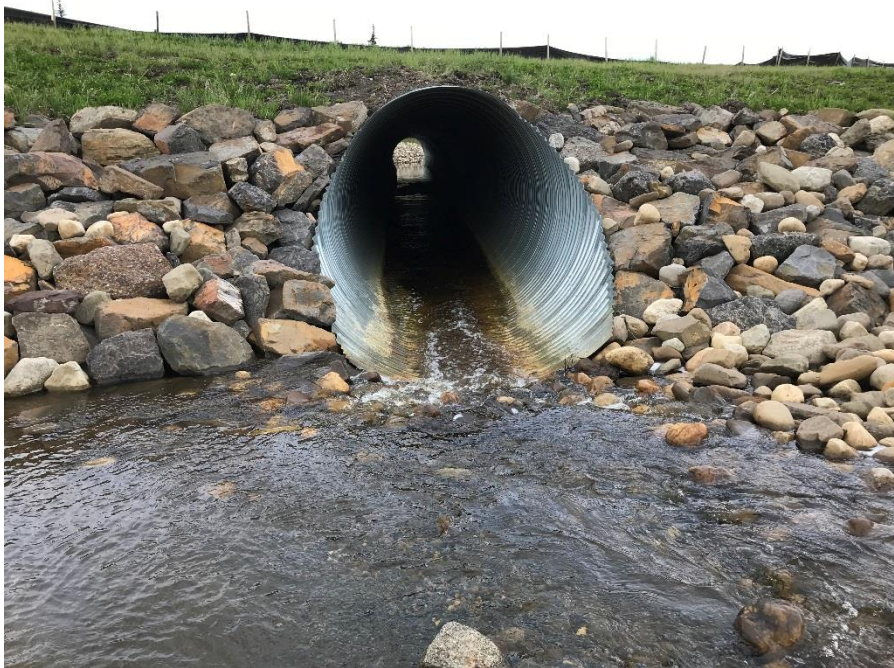
Photo 7: Culvert BF76754. Looking northeast.
