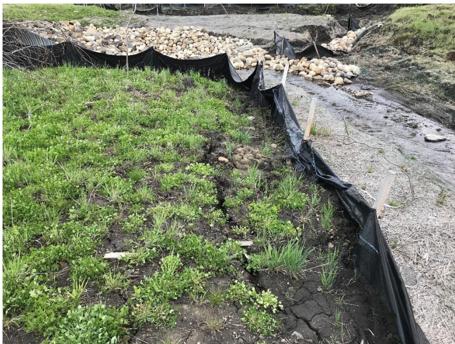
Photo 10: Tension crack about 100 mm wide southwest of BF76754. Looking east.
