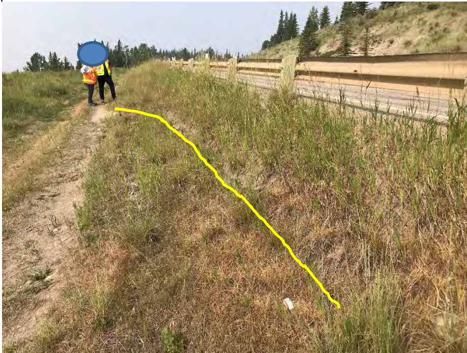
Photo 9: New scarp near “Hinton Entrance” sign. Looking west.
