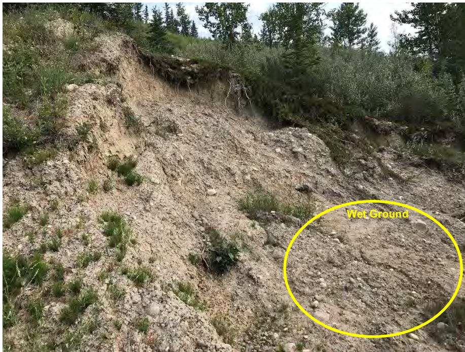
Photo 4: 1.5 m scarp with wet ground below access bench at west midslope slide. Looking north.
