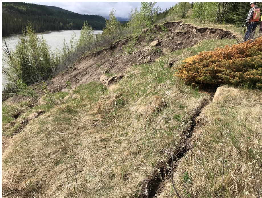
Photo 12: Between the two slides in Photos 7 and 8. Looking west.
