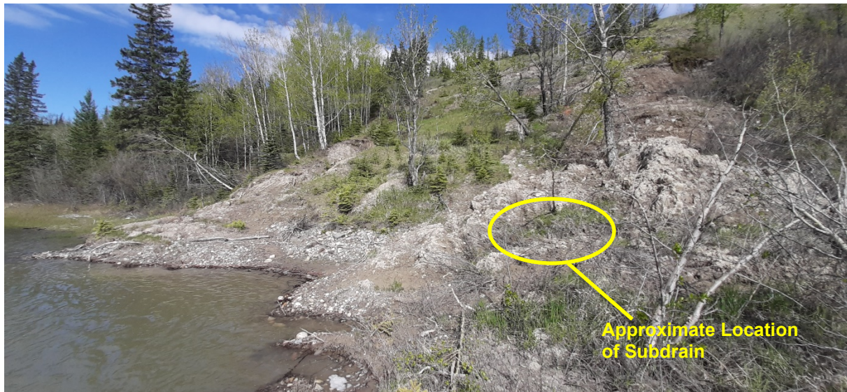
Photo 13: Overall Slope from toe. Looking northwest.
