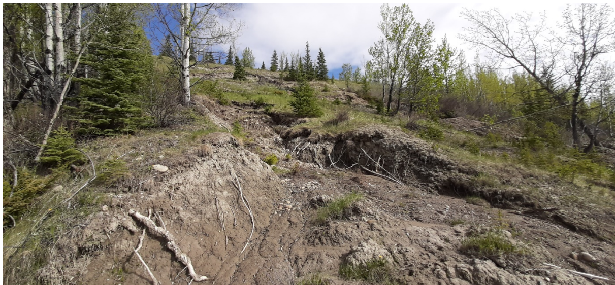
Photo 14: Overall Slope from toe. Looking north.
