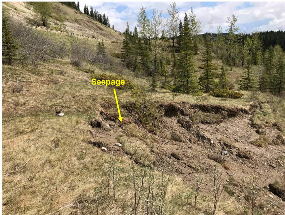
Photo 11: Slide about 20 m northeast of landslide in Photo 7. Seepage at base of scarp. Looking east.
