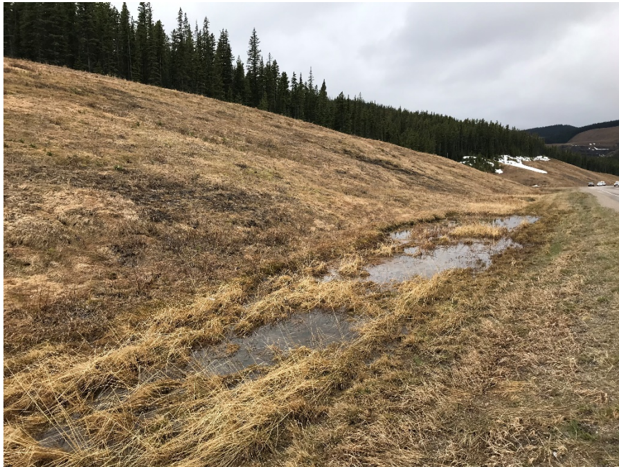
Photo 9: Skin slide south of Highway 40. Ponding in ditch. Looking southeast.
