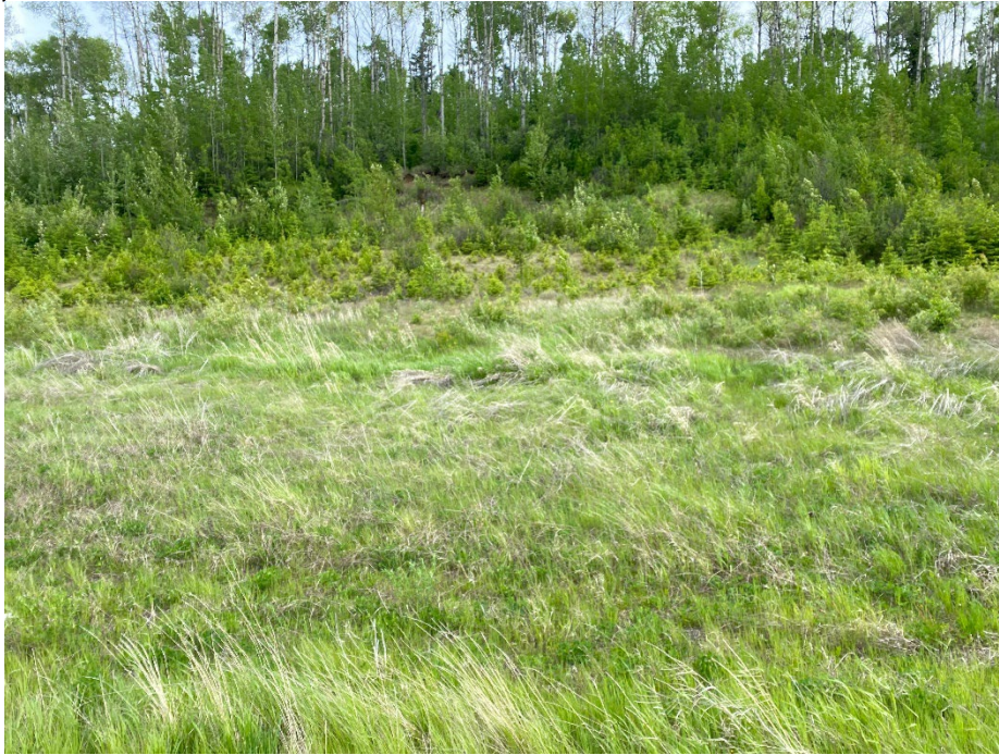
Photo 11: Scarp on south side of highway at approx. STA 34+700. Looking south.
