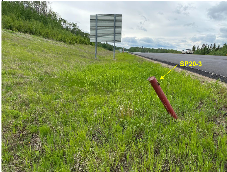
Photo 9: Repaired south slope and toe at approx. STA 34+875. Looking west.
