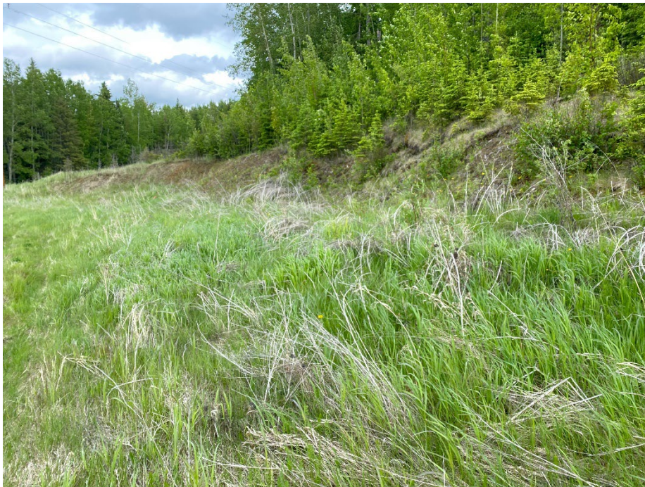
Photo 6: Increased vegetation on scarps. Old slumping on backslope. Looking southeast.
