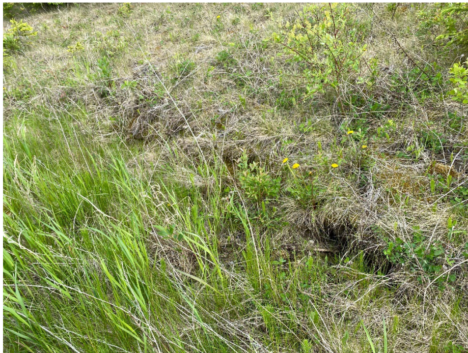
Photo 10: Cracking on slope near lower tree line, near STA 34+875. Looking southeast.
