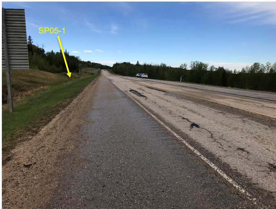
Photo 17: Highway condition at about Sta 34+675. Looking west.
