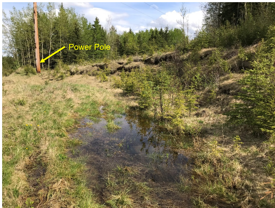
Photo 5: Fresh scarps and slumping on backslope. Ponding along base of scarp. Looking east.
