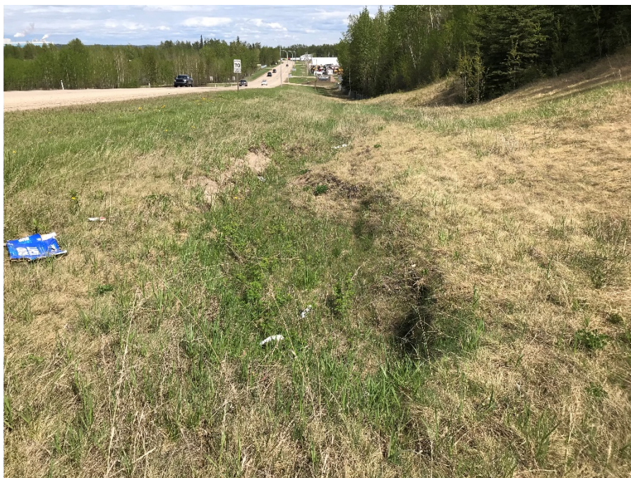
Photo 8: Erosion gully east of sign in Photo 6. Looking east.
