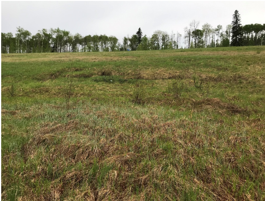
Photo 15: Tension crack/slump about 40 m west of Photo 12. Scarp up to about 1 m high. Looking south.
