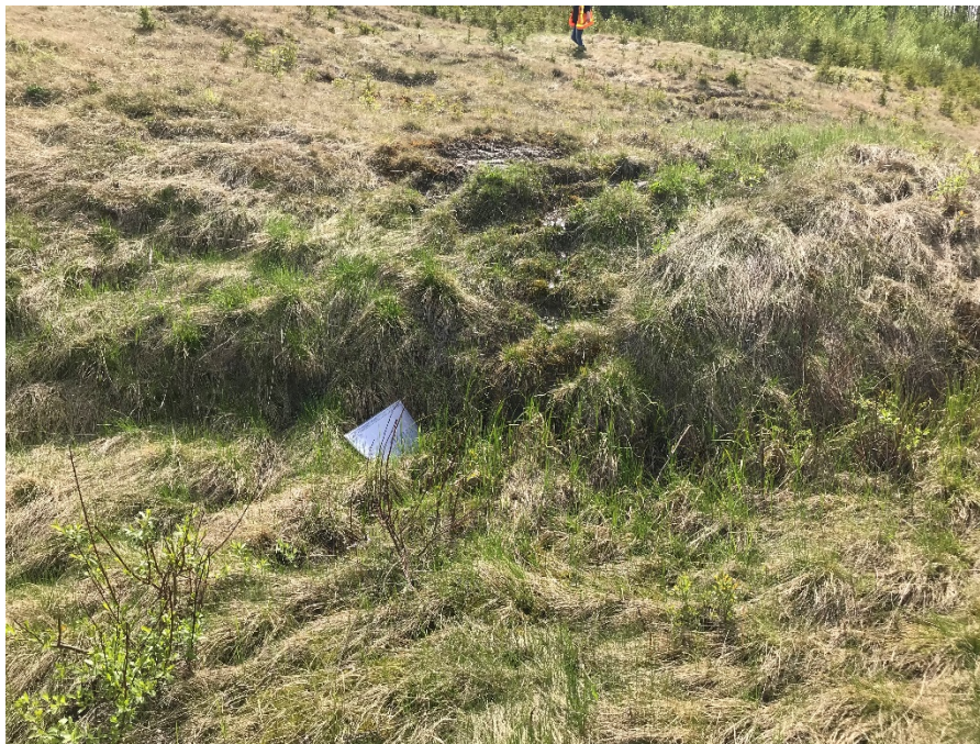
Photo 6: Potential spring or seepage with water flowing from top of toe bulge southeast of photoradar sign. Looking west.
