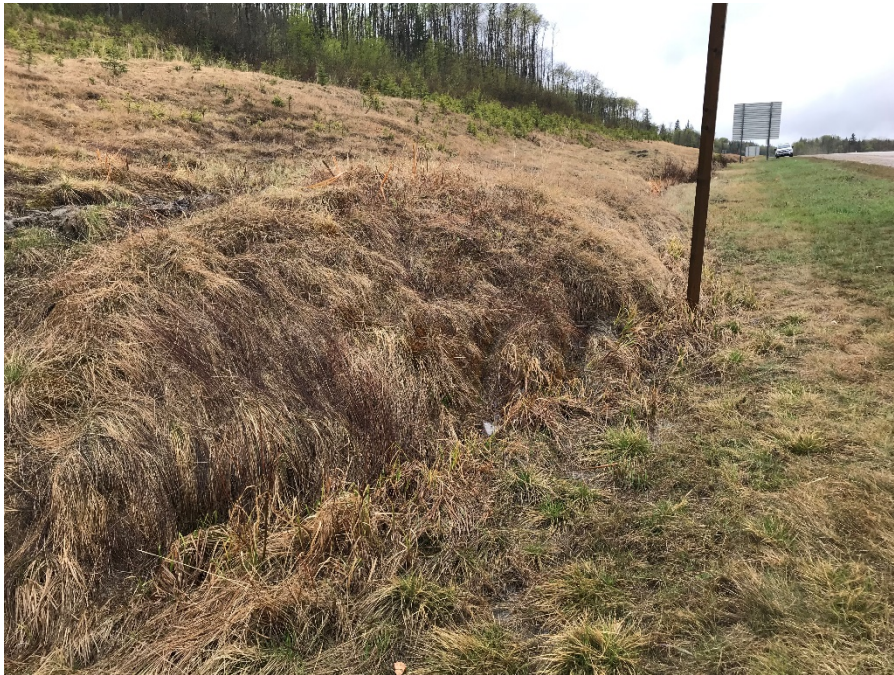
Photo 7: Toe bulge encroaching onto south ditch and sign post at Photo 6. Looking west.
