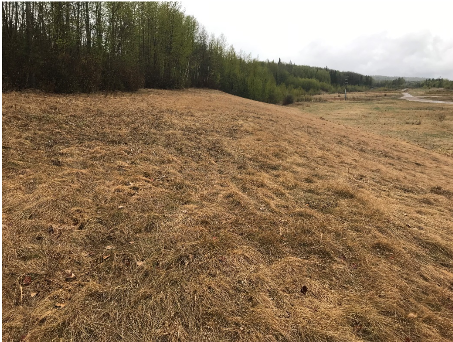
Photo 11: Overall view of lower toe berm. Looking west.
