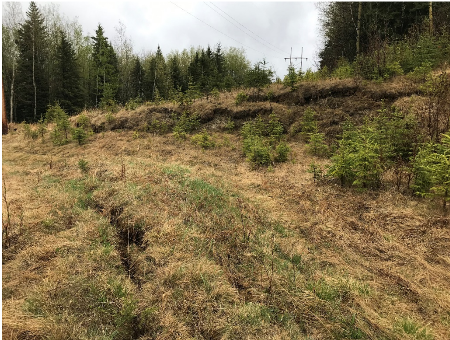
Photo 5: Fresh scarps with larger ground cracks west of the power pole south of the highway. Looking southeast.
