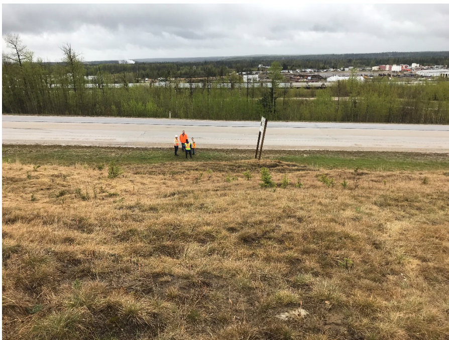
Photo 6: Leaning "Photo Radar" sign at power line site. Appears to be leaning more than previous inspection. Looking north.
