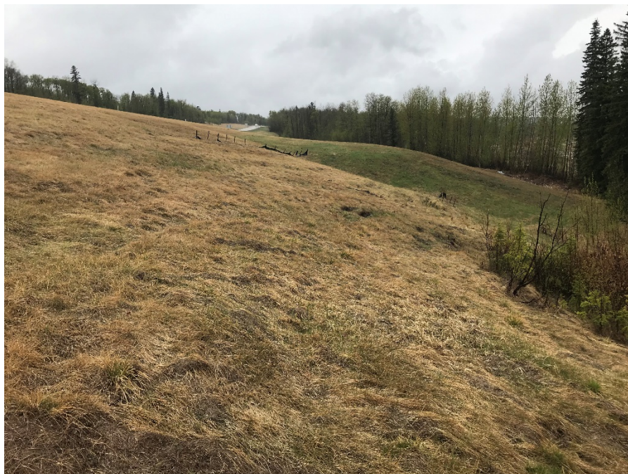
Photo 10: Overall view of upper toe berm. Looking west.
