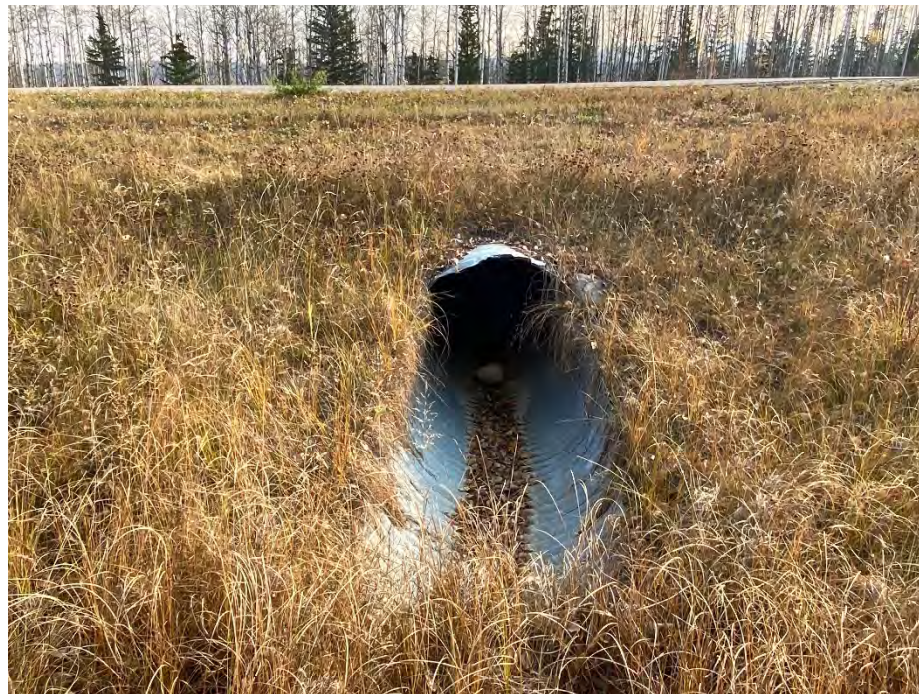
Photo 8: Culvert inlet, looking east.
