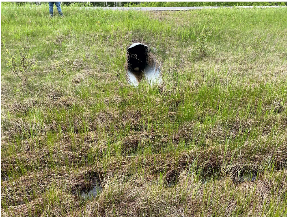
Photo 8: Culvert inlet and ponded water in ditch, looking east.
