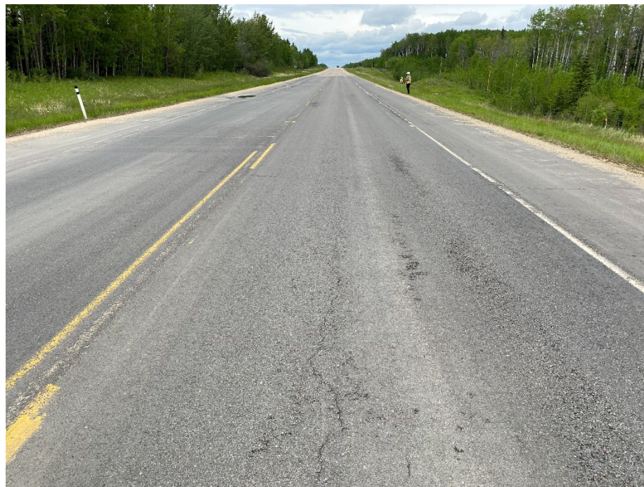
Photo 2: Pavement condition in NBL. Looking northeast.
