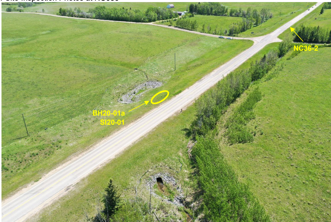
Photo 15: Site overview of NC036-1, taken by drone. Looking southeast.
