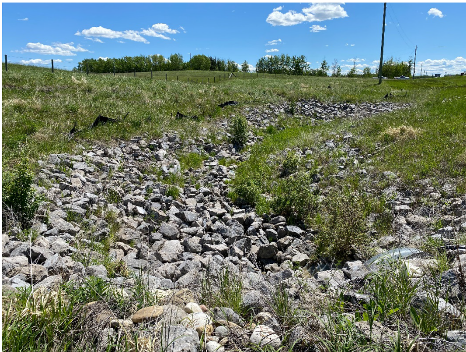
Photo 4: Riprap lined channel. Looking south.
