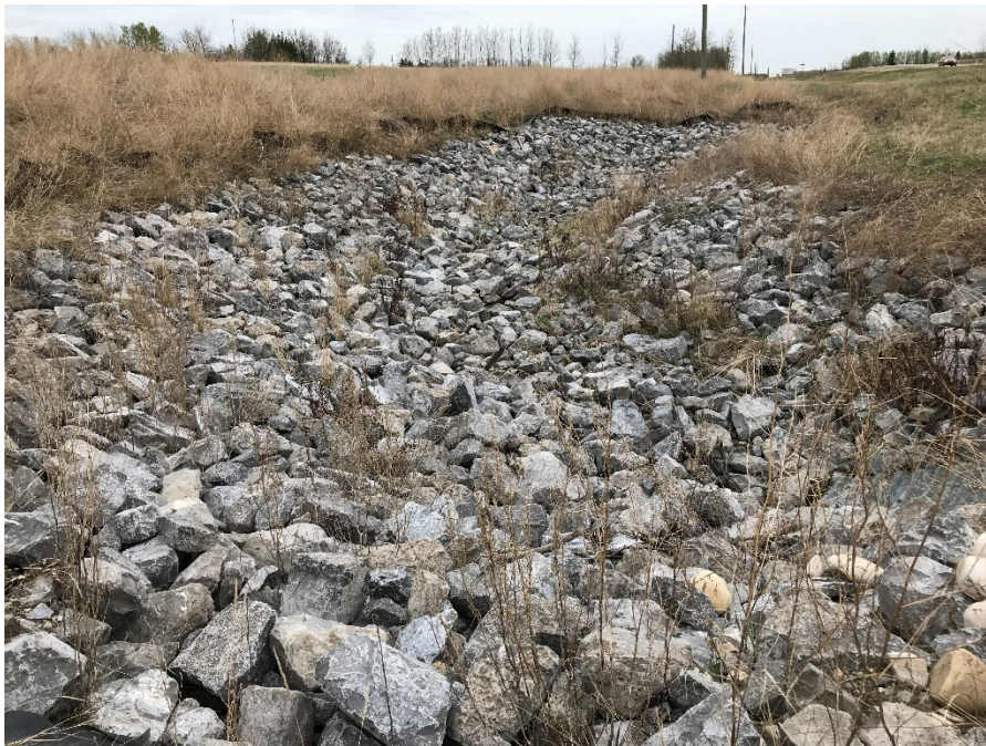
Photo 4: Culvert draining into riprap lined channel. Looking south.
