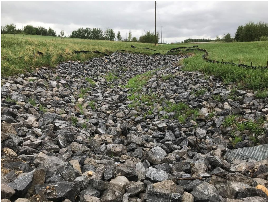
Photo 3: Culvert draining into riprap lined channel. Looking south.
