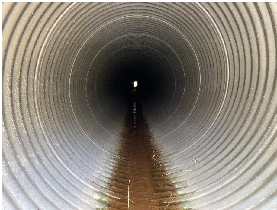
Photo 4: Culvert outlet. Looking southeast.
