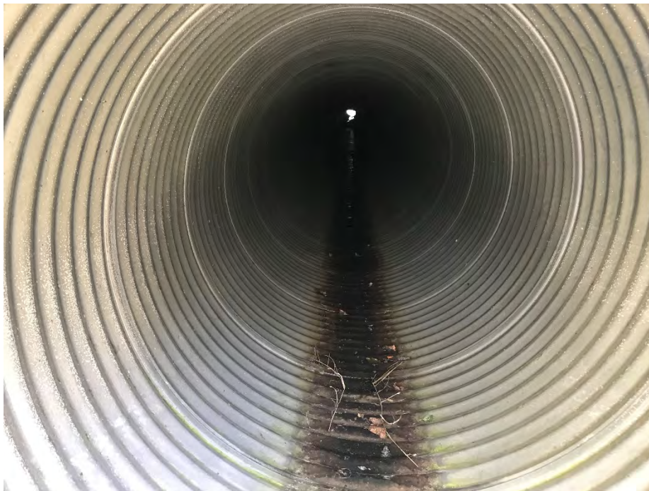
Photo 4: Culvert outlet. Looking southeast.
