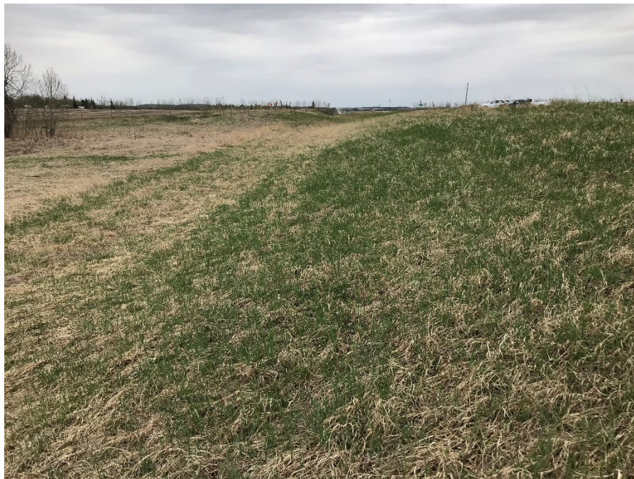
Photo 4: Overall west embankment slope. Looking north.
