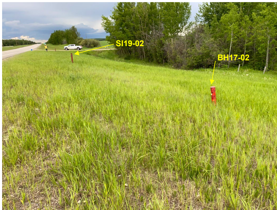
Photo 4: Slope inclinometers along pile wall on west embankment slope. Looking southwest.
