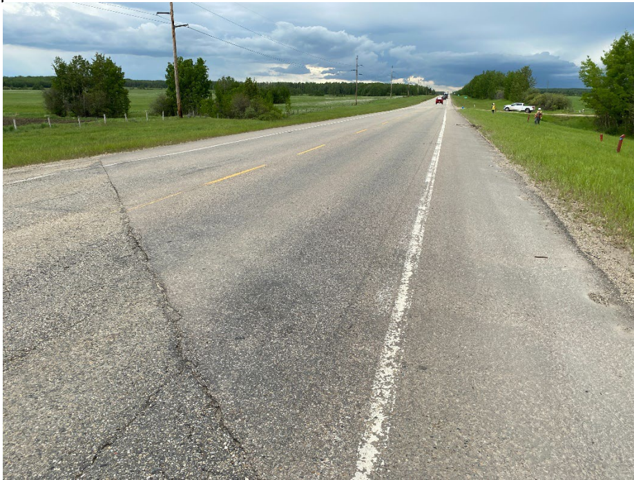
Photo 3: Pavement at north end of remediation limits. Looking south.
