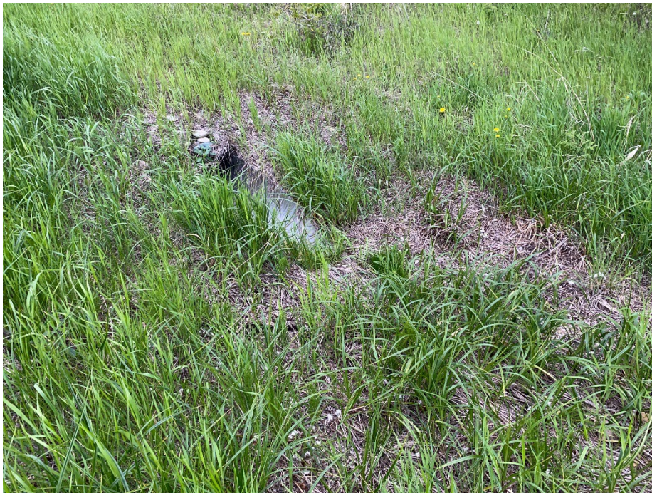
Photo 6: Culvert below driveway on west side of highway, looking southwest.
