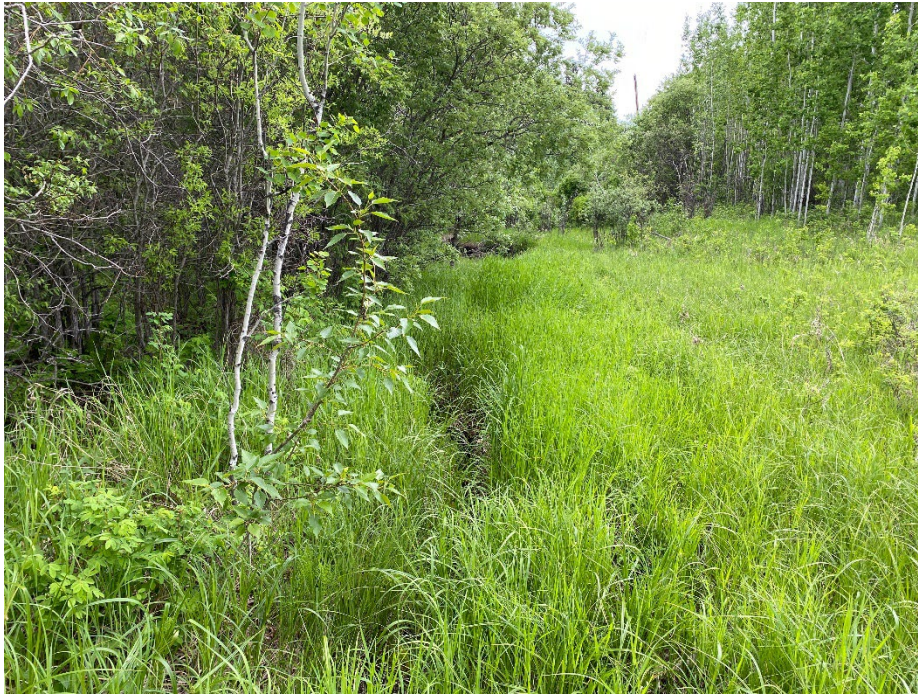
Photo 9: Flow from culvert leading from culvert outlet to erosion area. Looking north.
