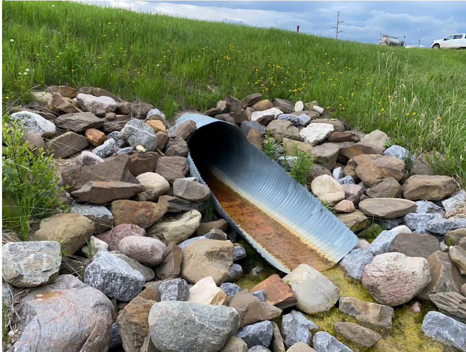
Photo 7: Culvert outlet on west side of highway. Looking southeast.
