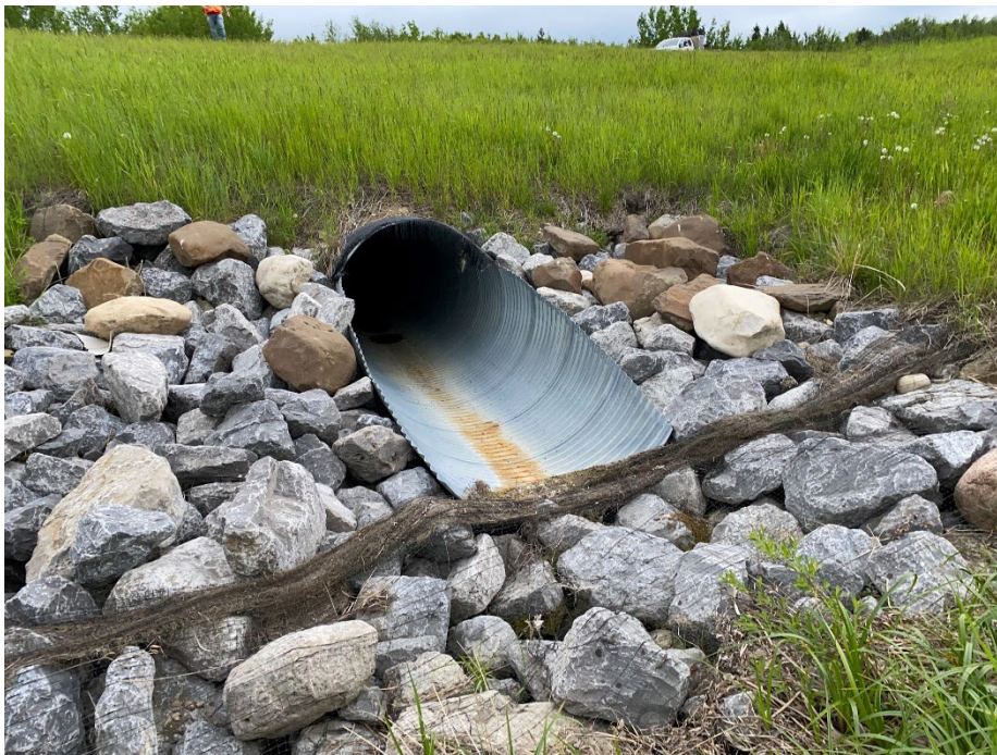
Photo 8: Culvert inlet on the east side of the highway. Looking northwest.
