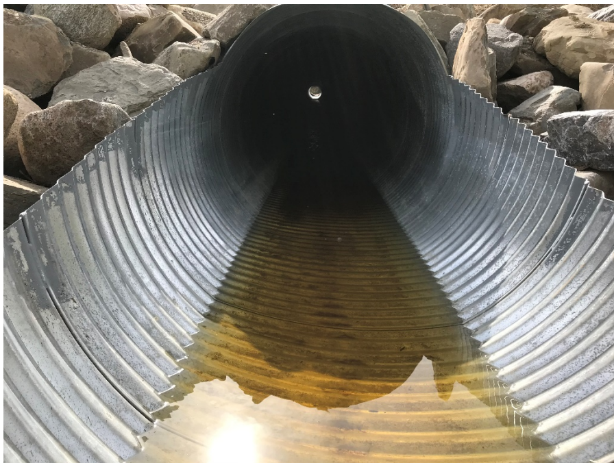
Photo 8: Culvert condition from outlet. Looking southeast.
