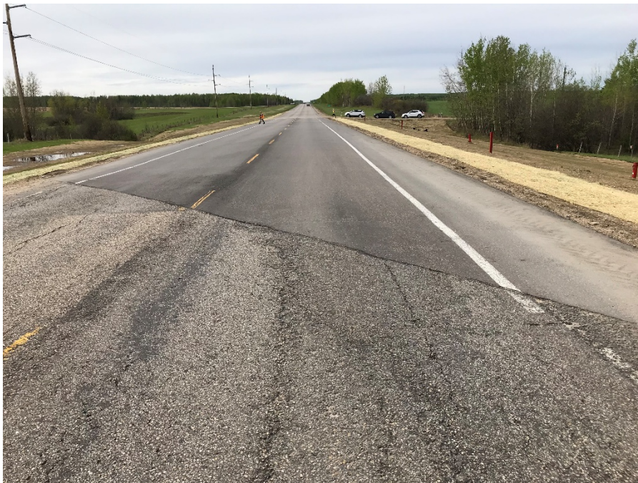
Photo 1: Reconstructed pavement at north end of remediation limits. Looking south.
