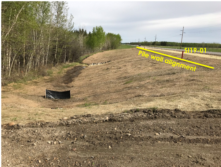
Photo 9: Overall repaired west embankment slope. Looking north.
