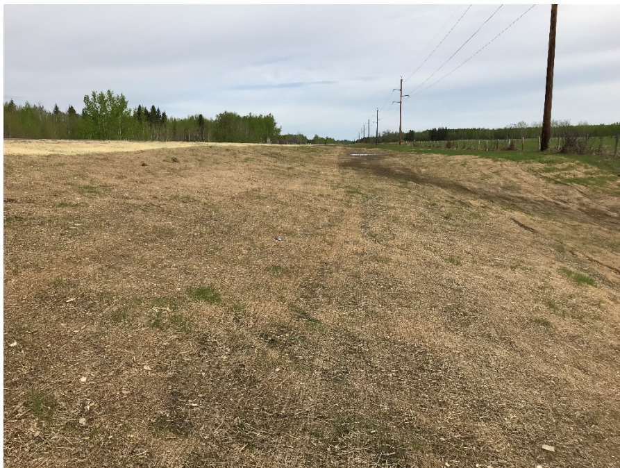
Photo 10: Overall east embankment slope. Looking north.
