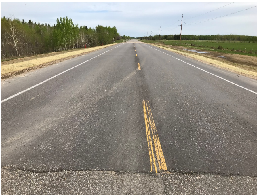
Photo 2: Reconstructed pavement at north end of remediation limits. Looking south.
