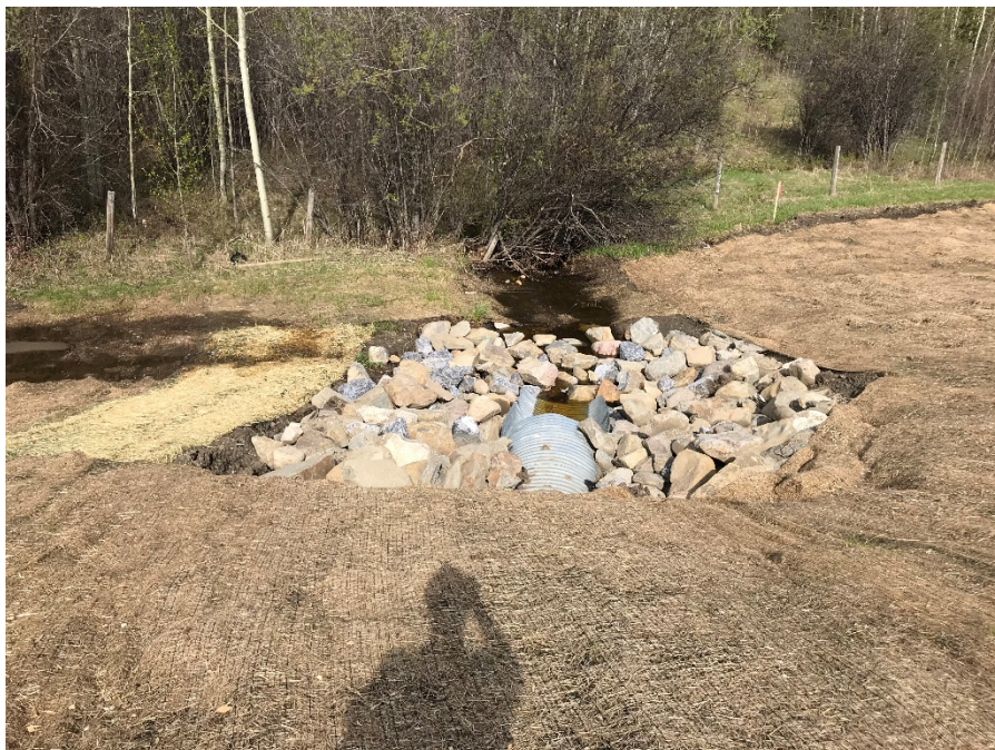
Photo 6: Culvert outlet. Looking northwest.
