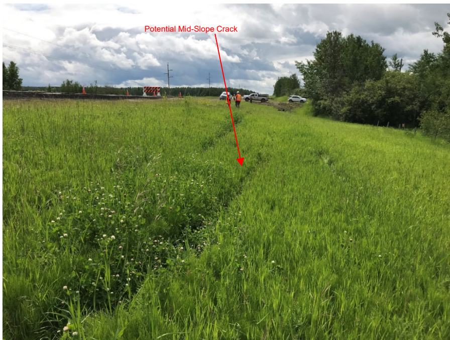
Photo 10: Looking south at the mid-slope. Note potential mid-slope crack. The foot track was created during locating the potential mid-slope crack. Photo taken July 11, 2019.
