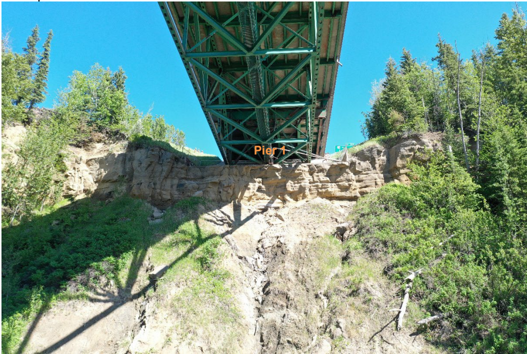
Photo 3: Sandstone outcrop and gullies downslope of east abutment, facing east.
