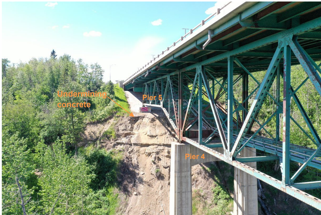
Photo 8: West abutment and riverbank, facing northwest.
