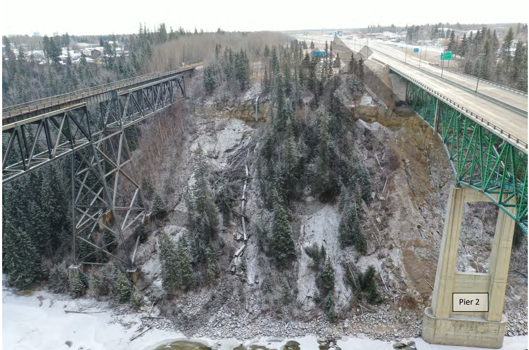
Photo 1: Overview of northeast slope, facing east
