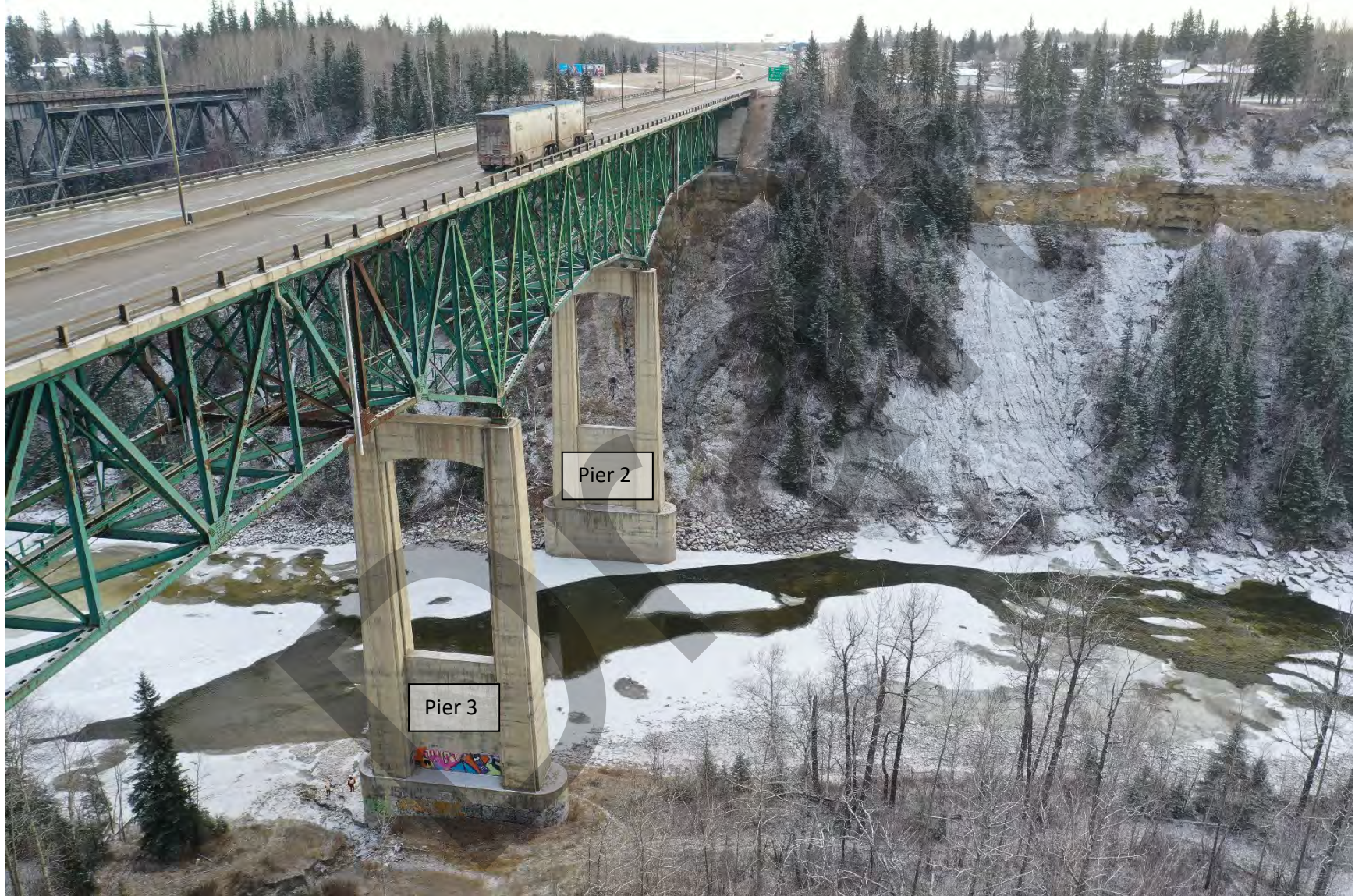
Photo 2: Overview of southeast slope, facing east
