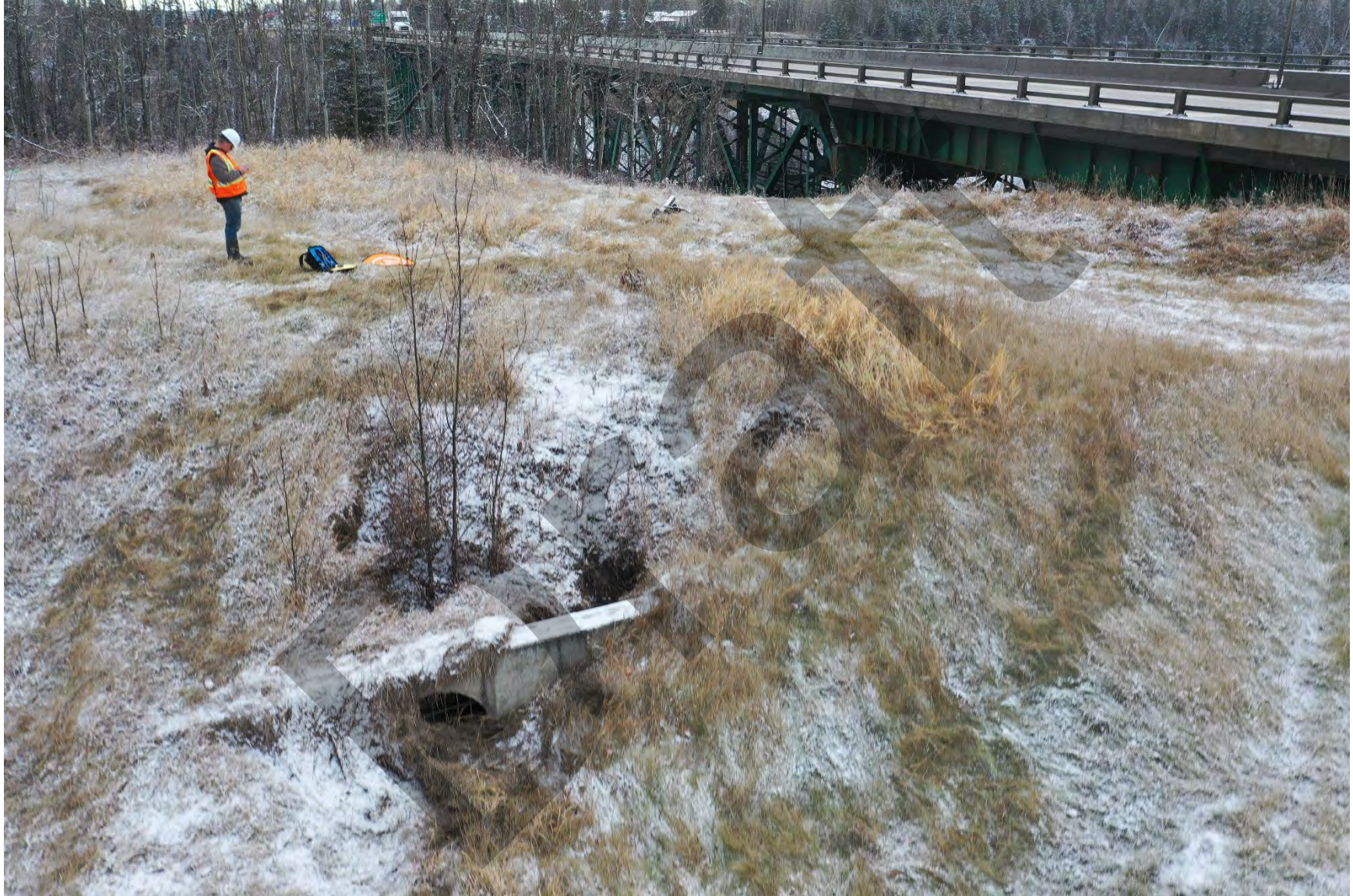
Photo 19: Entrance to culvert north of west abutment, facing east
