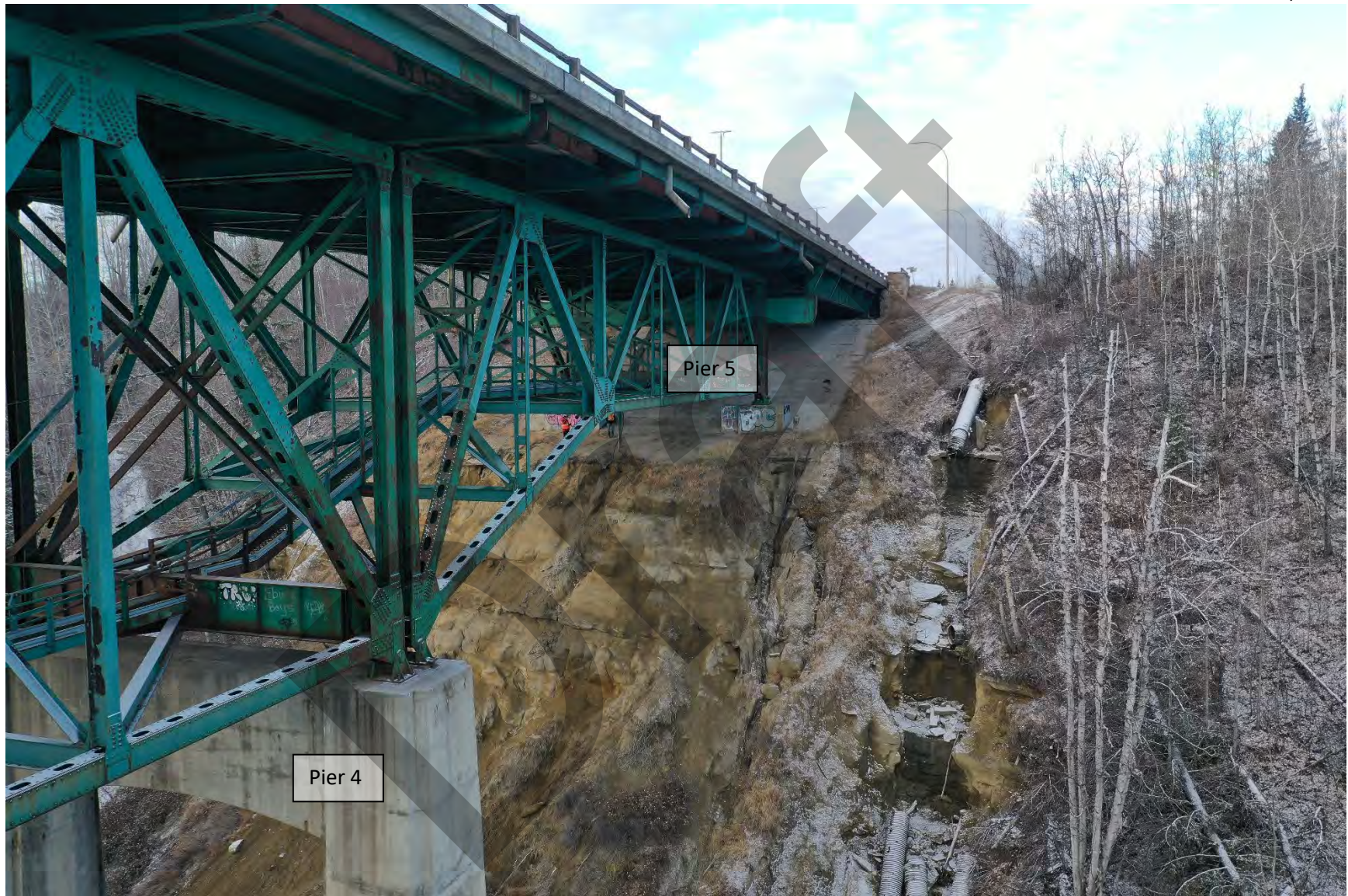
Photo 17: Erosion at west abutment slope, facing west, showing broken sections of culvert and erosion gullies
