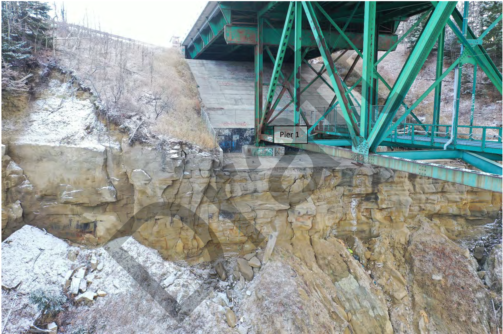
Photo 5: Slope face next to east abutment, facing east
