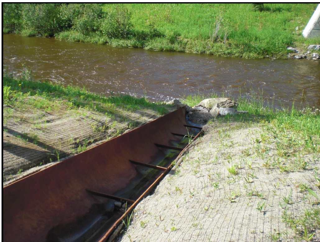
PHOTO 9: Half round culvert installed in 2012.
