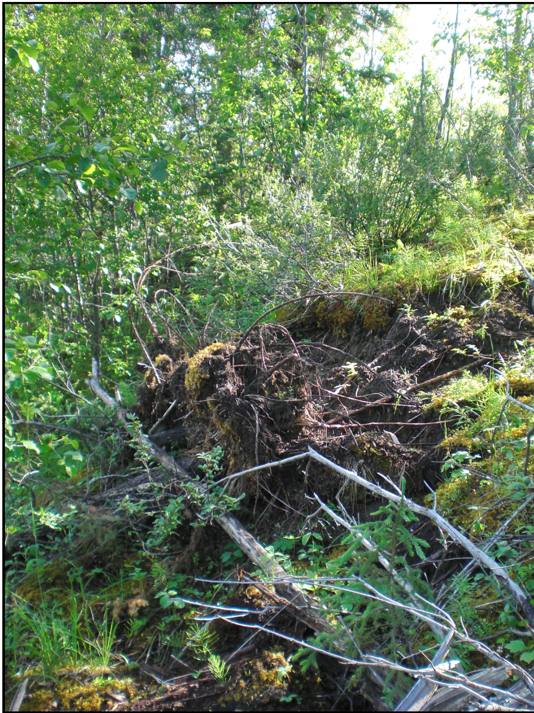
PHOTO 2: Freshly exposed earth in scarps south of pile wall.
