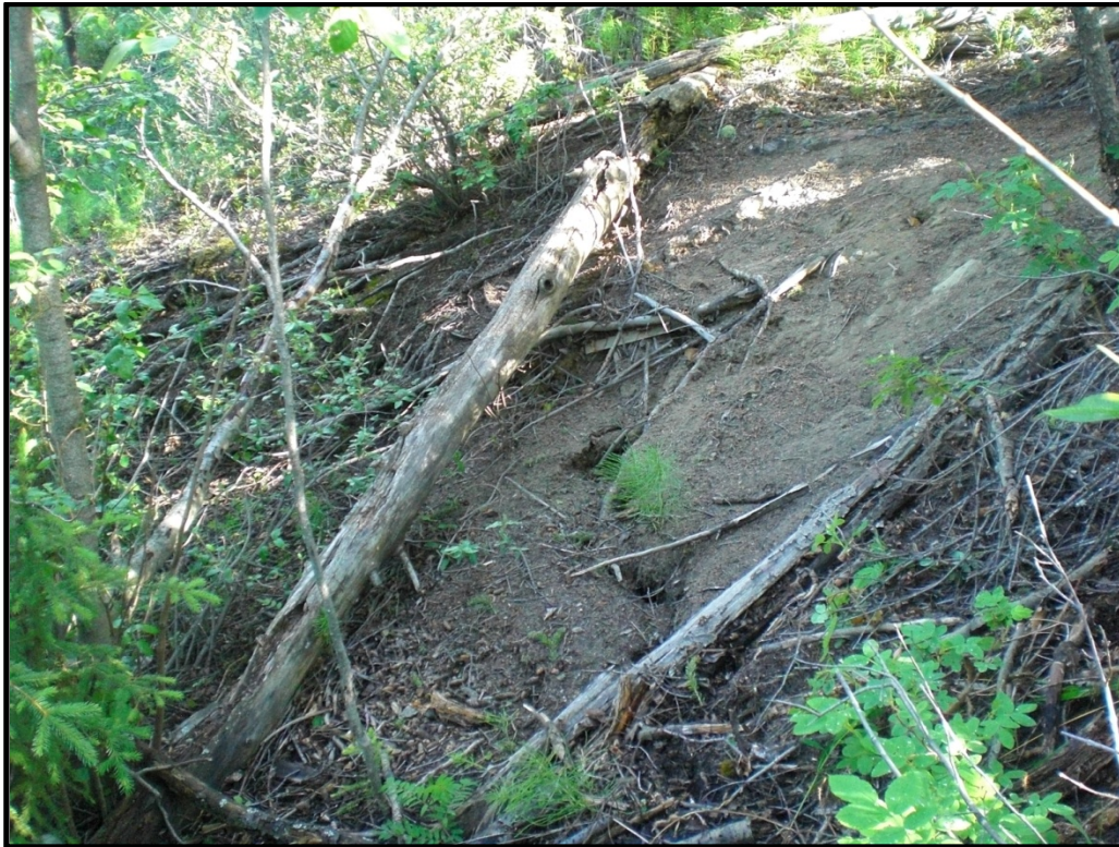
PHOTO 4: Tension cracks in slope below crack south of pile wall.
