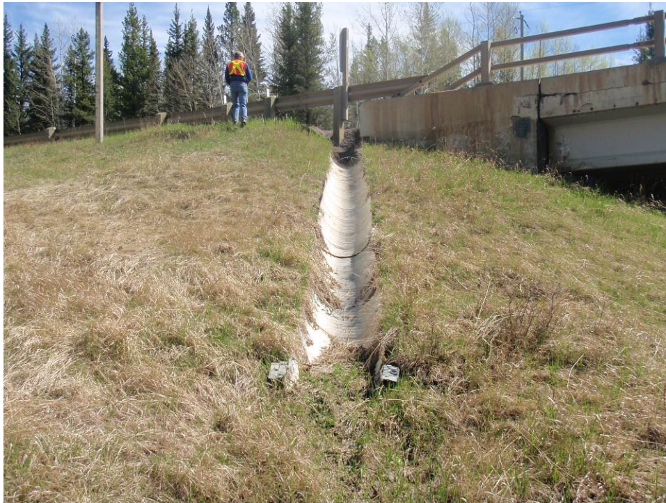
Photo 9 – Half round down drain at NW bridge quadrant (May 17, 2011).
