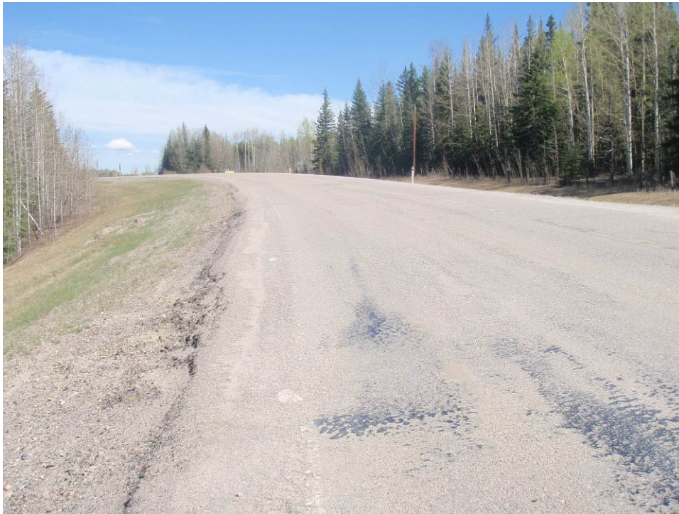
Photo 1 – Looking north at roadway above repaired side slope (May 17, 2011).
