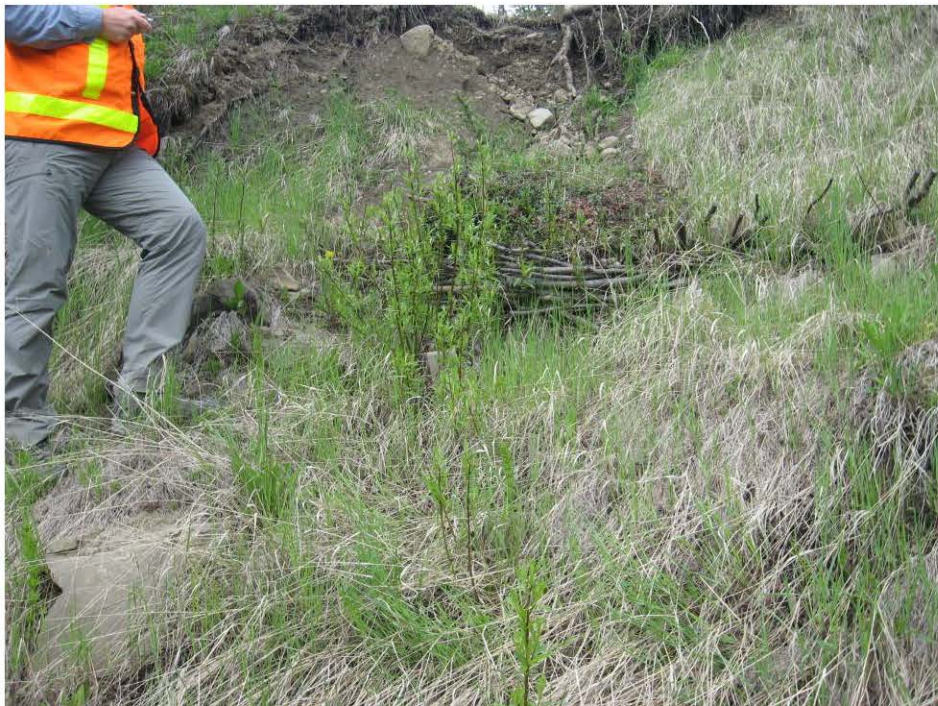
Photo 10 – Modified Brush Layering with Wattles (furthest upstream) showing one season's growth and minor slumping at top, June 12, 2008.
