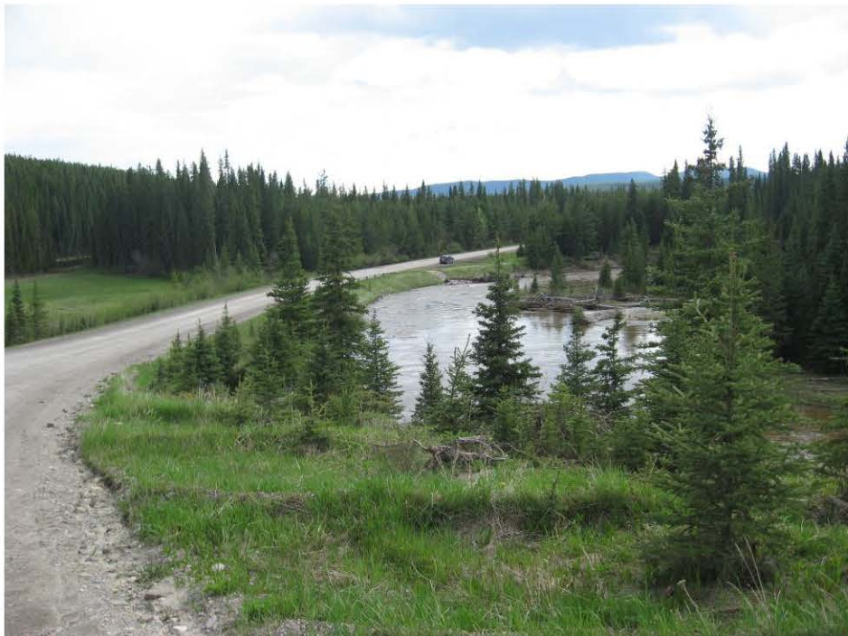
Photo 2 – Looking southeast at repaired main slump area, June 12, 2008.
