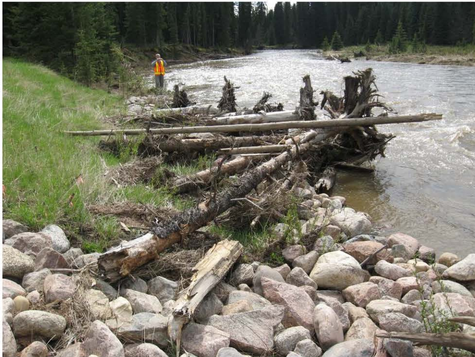
Photo 4 – View of displaced rootwads at upstream end of treatment, June 12, 2008.
