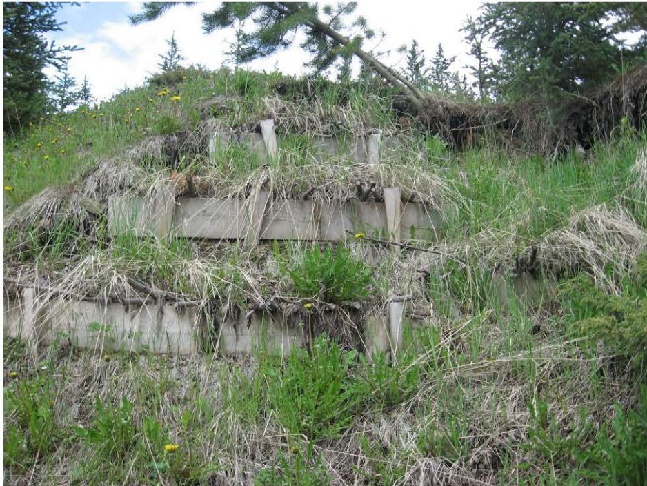
Photo 9 – Modified Brush Layering with Cedar Boards, June 12, 2008.
