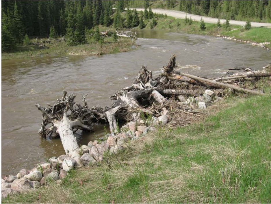
Photo 3 – Looking upstream at rootwads. Note that upstream 2 have shifted, June 12, 2008.
