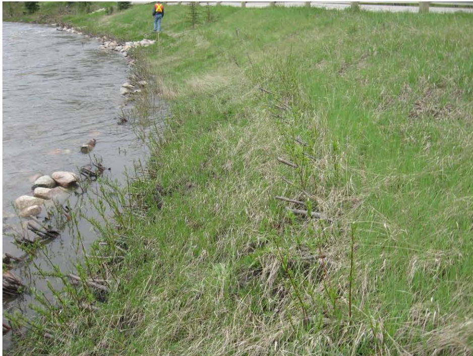
Photo 1 – Looking northeast at repaired slump area below guardrail, June 12, 2008.
