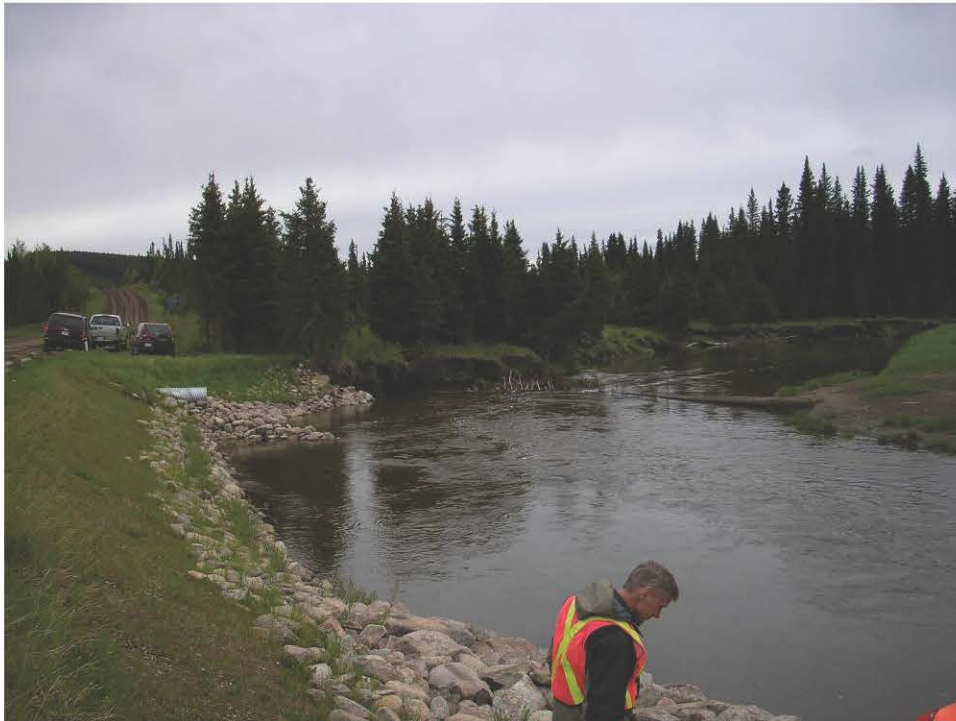
Photo 1 – Looking east (downstream) at culvert and Vane 4, June 12, 2007.
