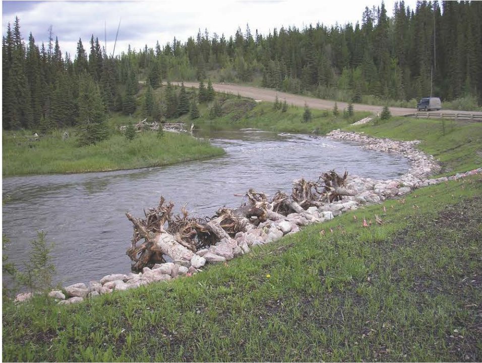
Photo 3 – Looking north at north slope area, June 12, 2007.
