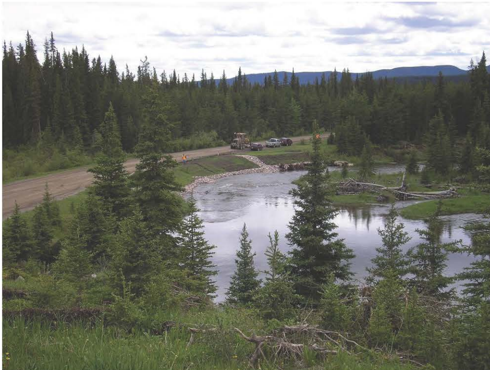
Photo 2 – Looking southeast at repaired main slump area, June 12, 2007.
