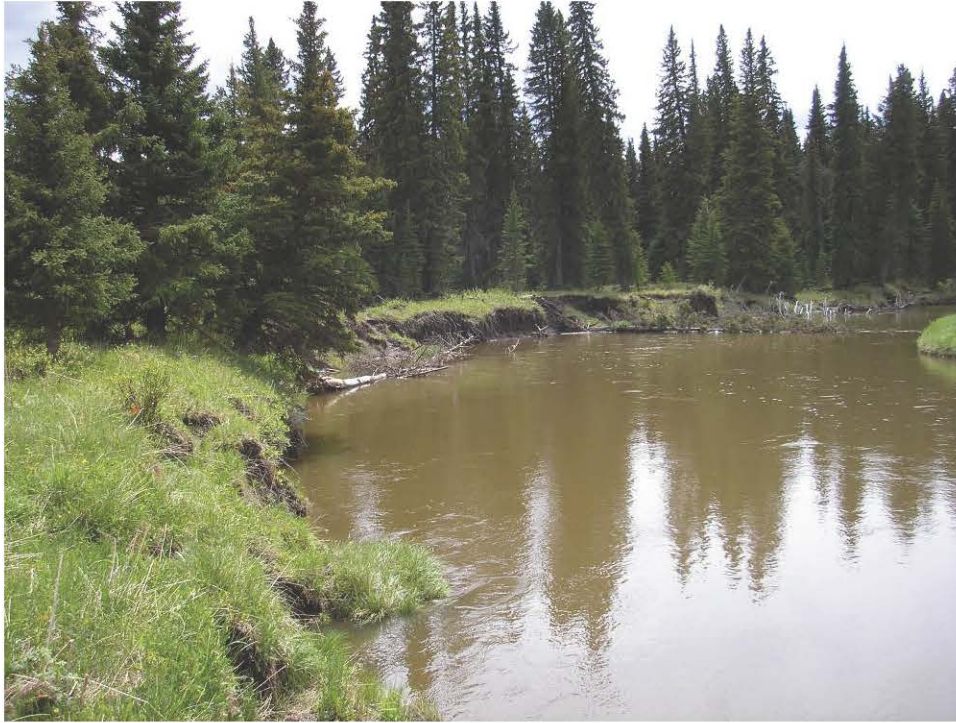
Photo 3 – Looking at eroding outside bank downstream of Site 9, June 12, 2007.
