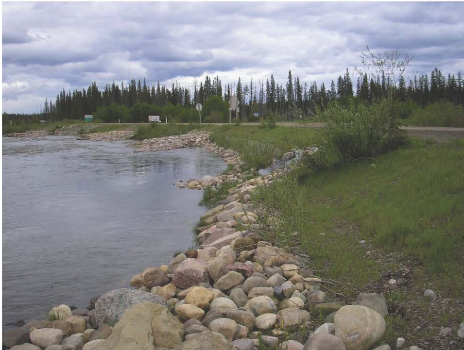
Photo 3 – Looking east (downstream) at culvert and Vanes 4 to 6, June 12, 2007.
