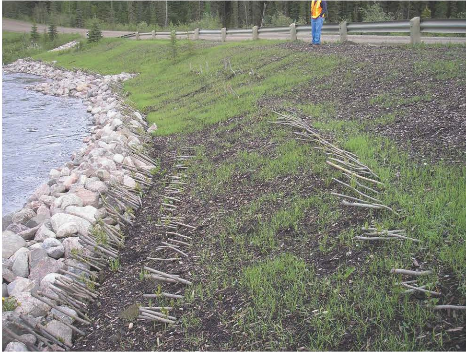
Photo 1 – Looking northeast at repaired slump area below guardrail, June 12, 2007.
