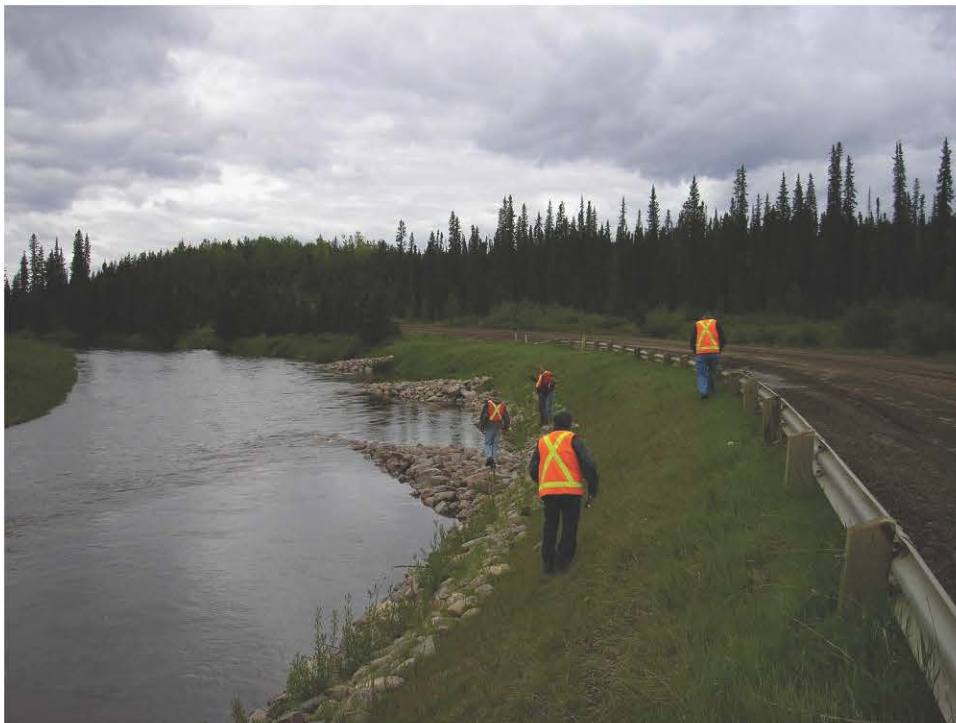
Photo 2 – Looking west (upstream) at Vanes 3, 2, and 1, June 12, 2007.
