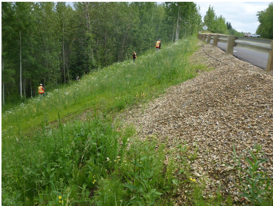
Photo 4: Overall view of the repaired slope. Looking east.
