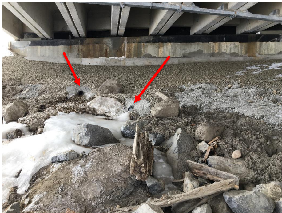
Photo 4: Two new subdrains installed in west abutment. Looking west.
