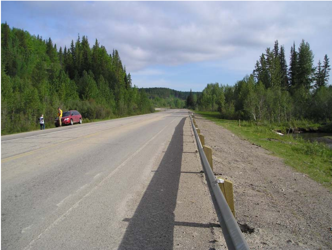
Photo 3 – Looking north along edge of pavement.
