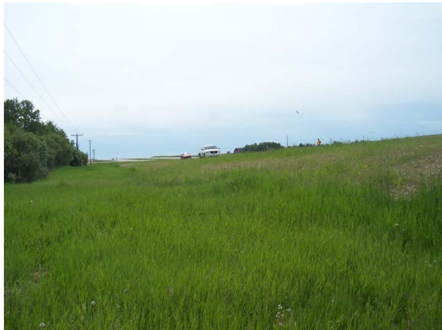
Toe berm looking southeast.
