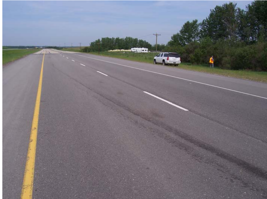
Northbound lane – No pavement distress.
