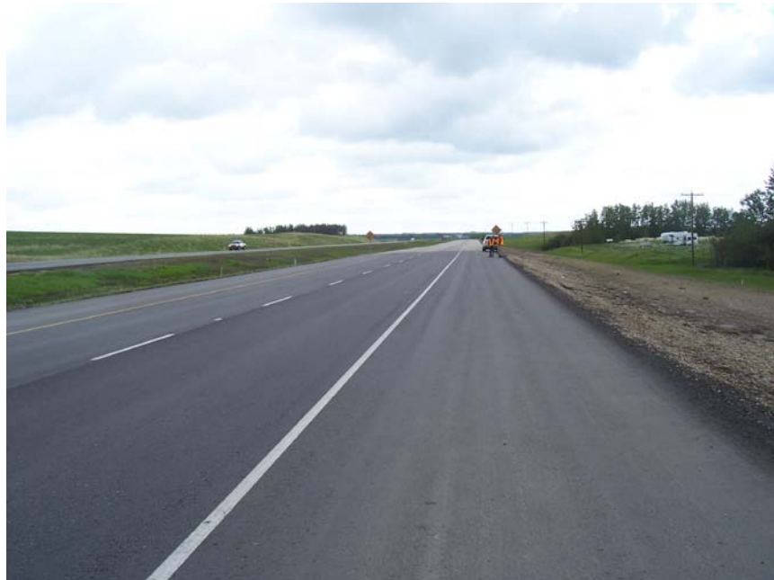
Photo 1 – New pavement overlay.
