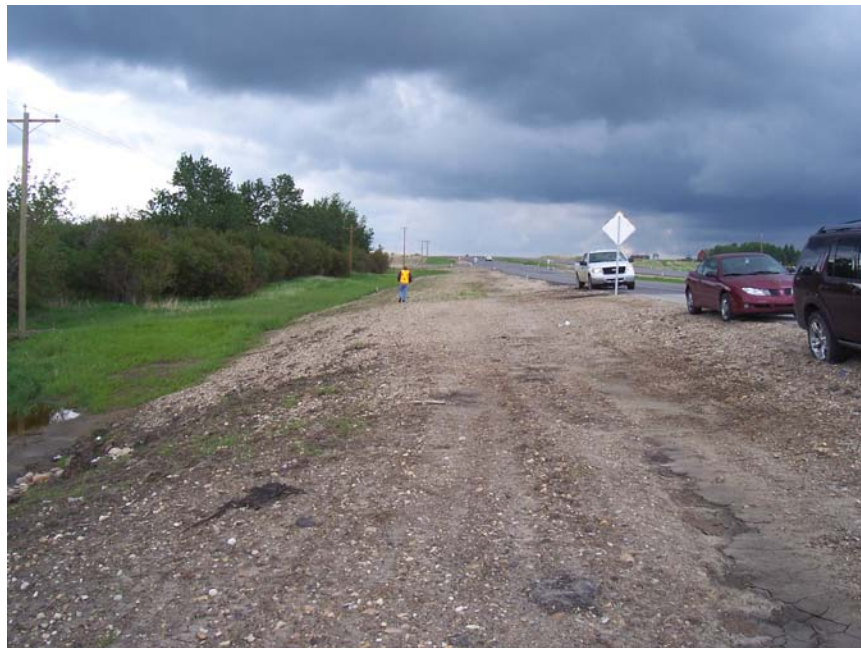
Photo 2 – New toe berm.
