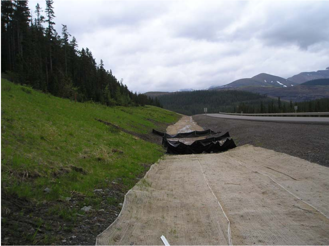
Photo 3 – East ditch (looking south, culvert inlet in foreground) June 1, 2005
