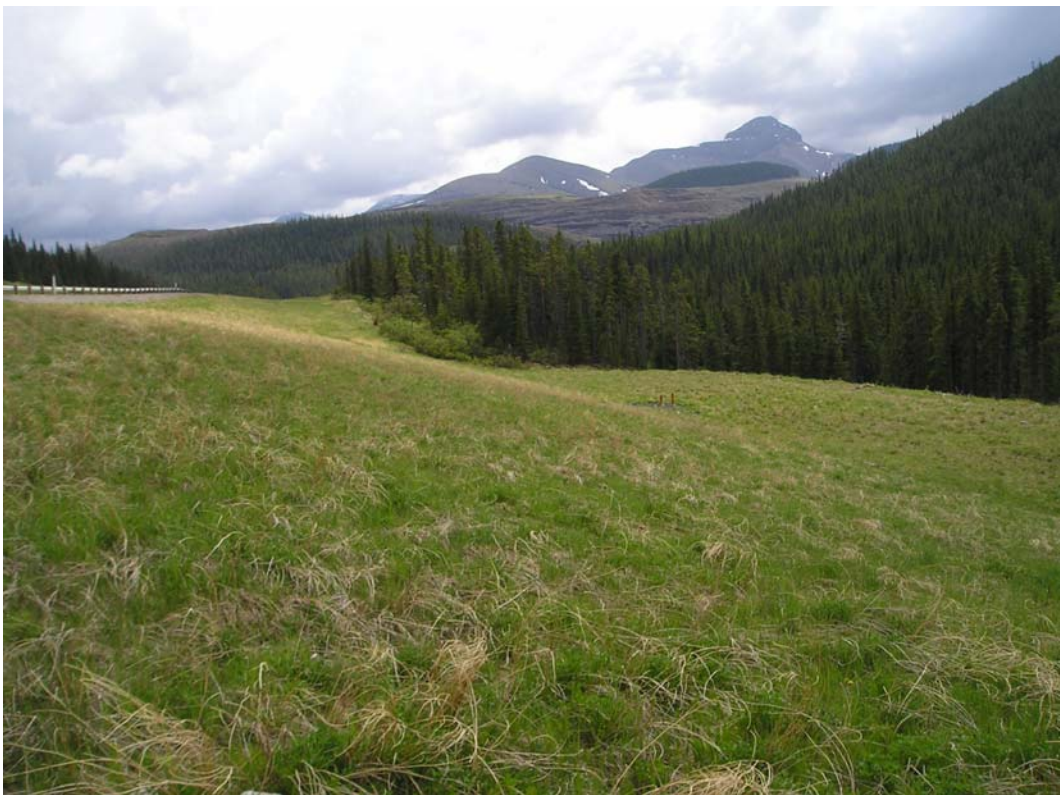
Photo 2 – Looking south at repaired side slope.
