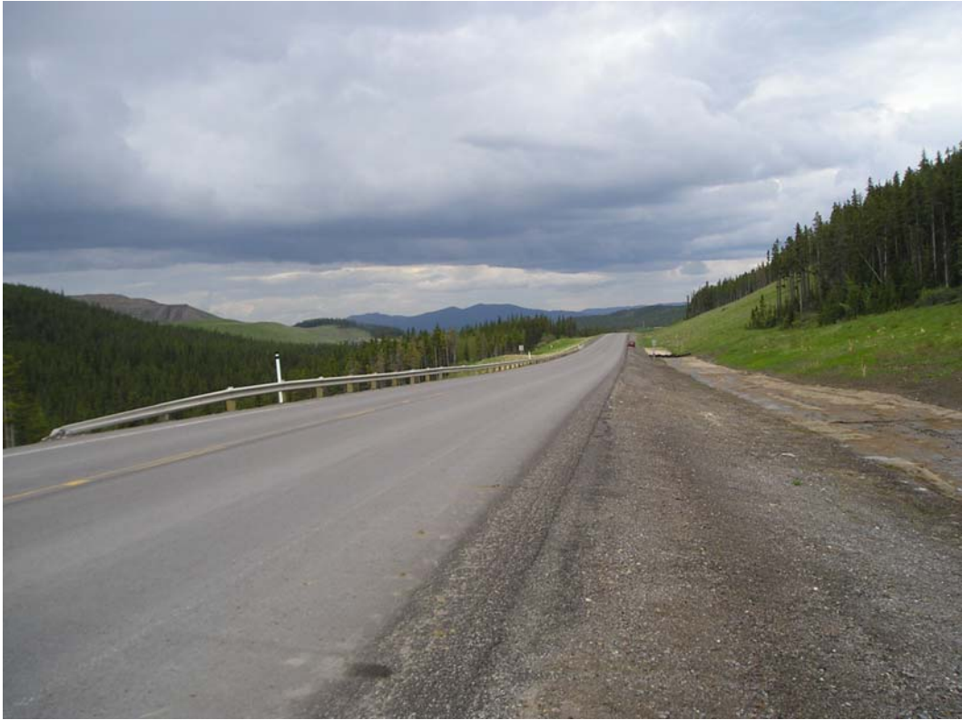
Photo 5 – East ditch and pavement surface (looking north). June 1, 2005
