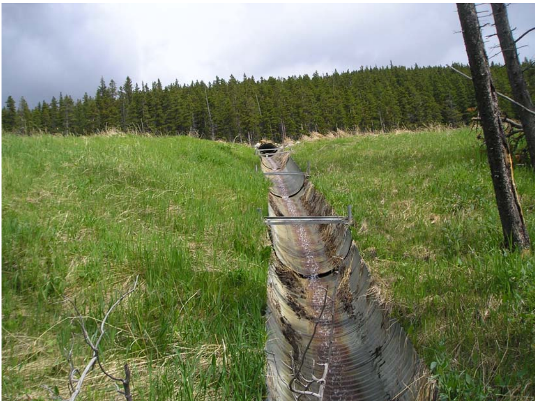
Photo 6 – Half round culvert flow from east ditch (looking east) June 1, 2005
