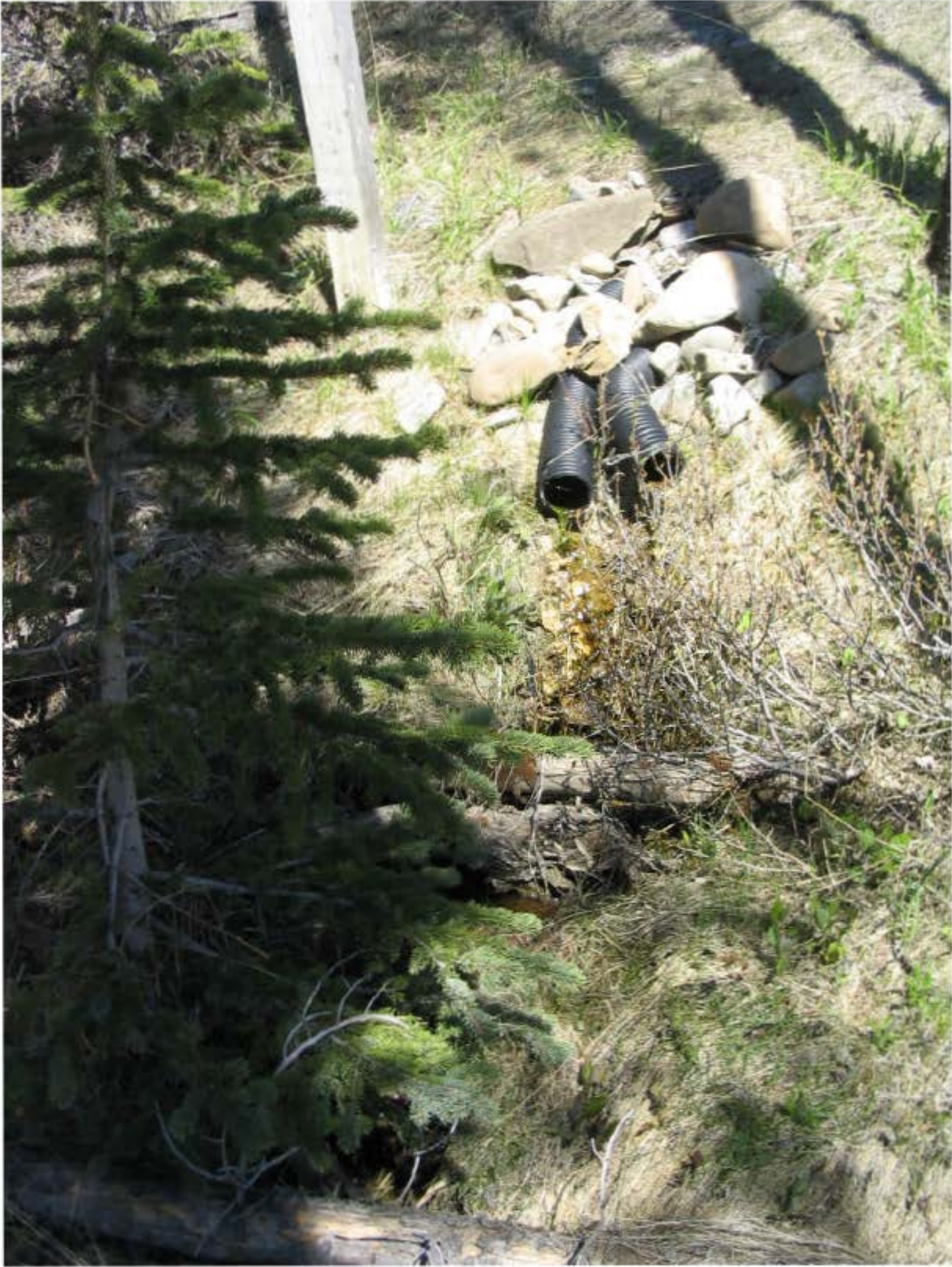
PHOTO 6 - 1990 SUBDRAIN OUTLET (LOOKING EAST)
