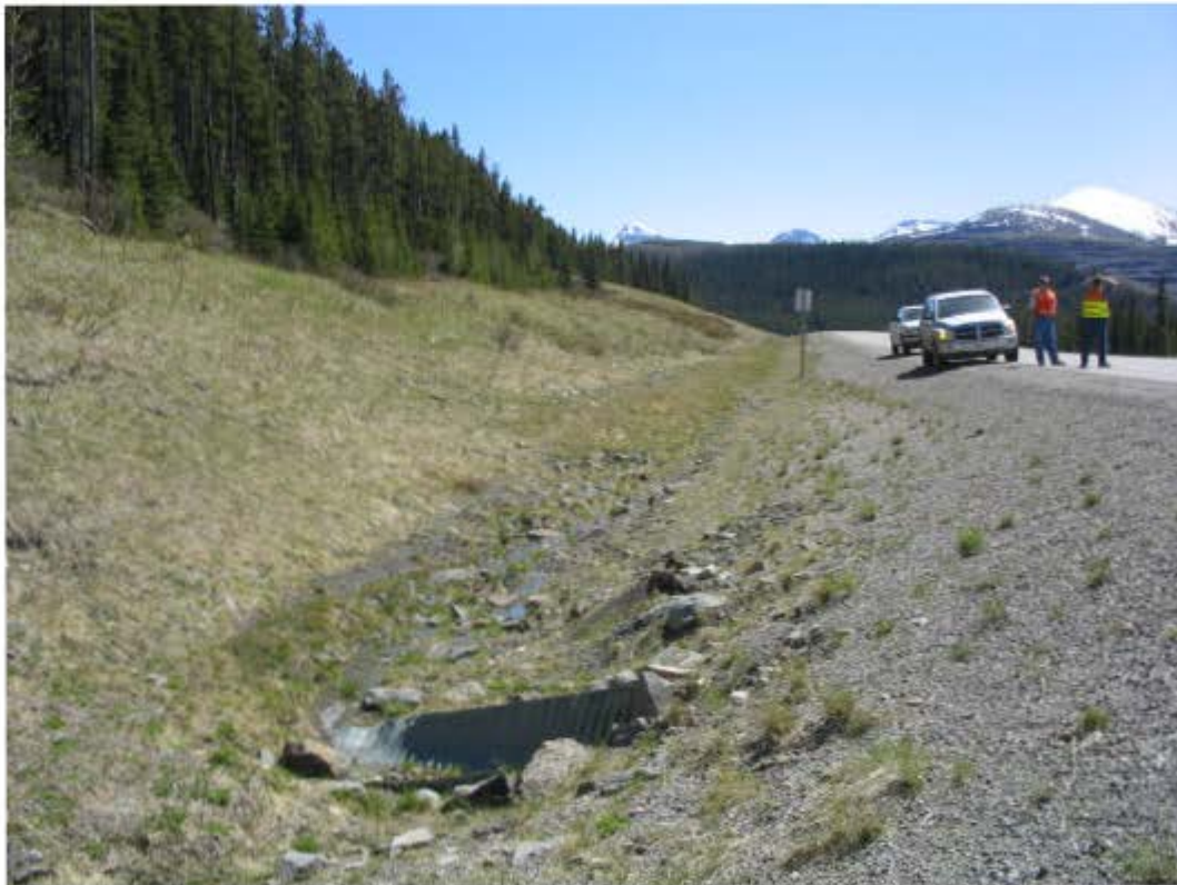
PHOTO 3 - EAST DITCH LOOKING SOUTH (CENTERLINE CULVERT INLET IN FOREGROUND)
