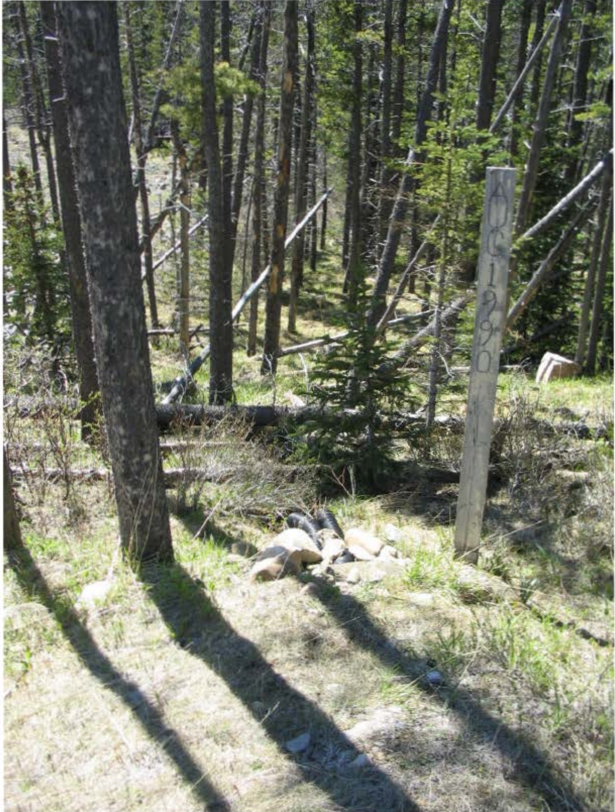
PHOTO 5 - 1990 SUBDRAIN OUTLET (LOOKING WEST)
