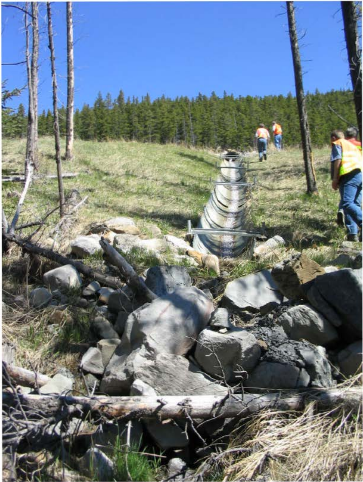
PHOTO 8 - HALF ROUND CULVERT FLOW FROM EAST DITCH ( LOOKING EAST)
