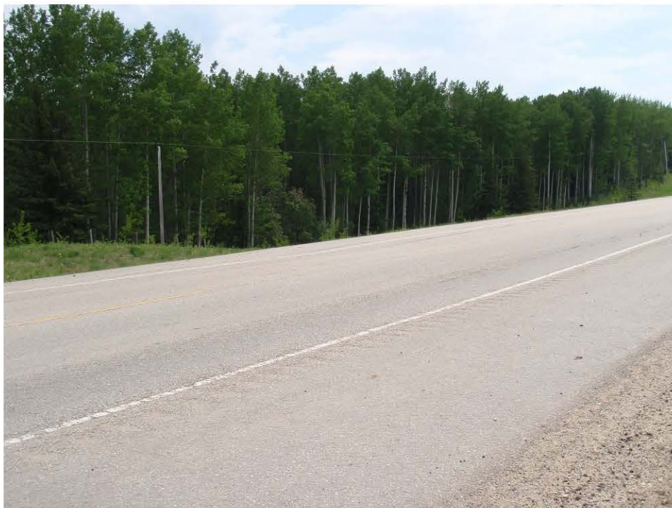
Photo 2 – Looking south at Dip 2.
