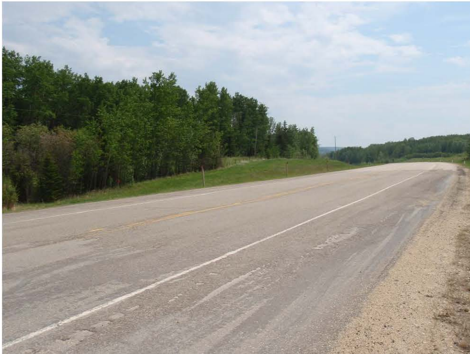
Photo 5 – Looking south at patch over Dip 3.
