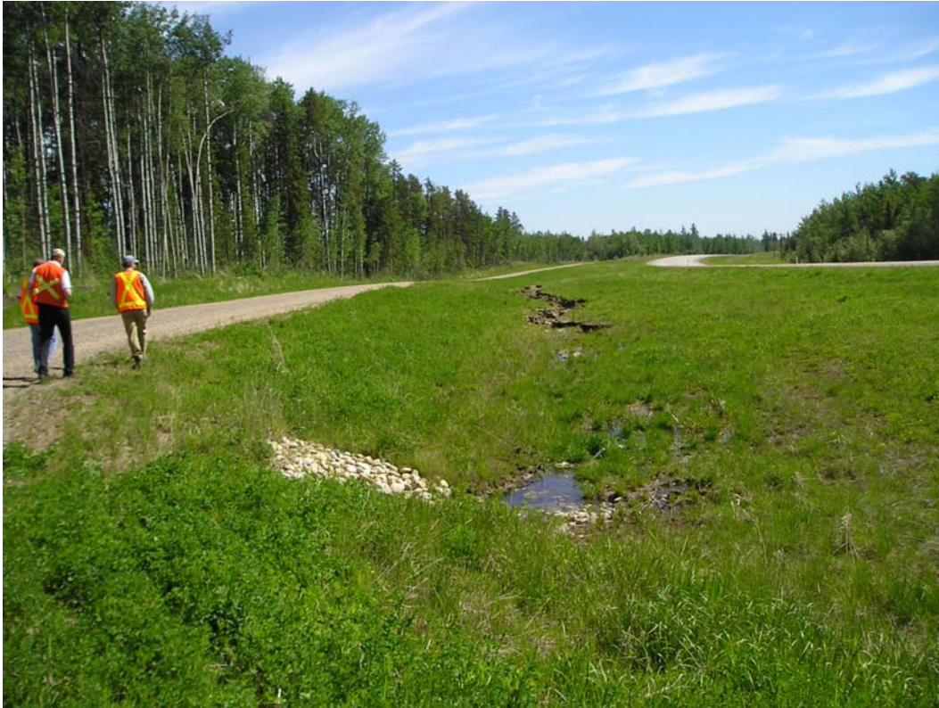
Photo 1 – Looking east from 800 mm dia CSP outlet. May 31, 2005
