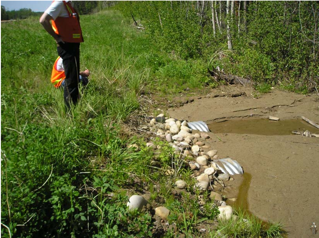
Photo 4 – Twin culvert outlet area (looking west).
