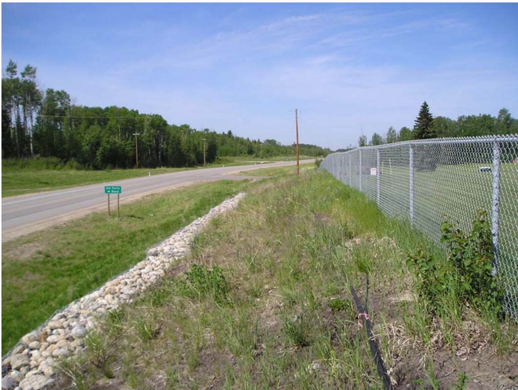
Photo 2 – Looking west at area behind wall (Telus line in foreground).
