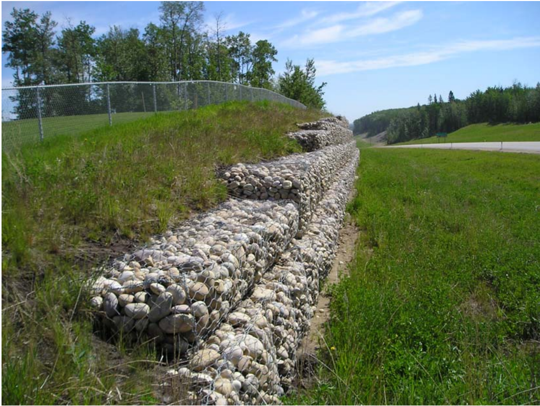
Photo 1 – Looking east at west end of gabion wall.
