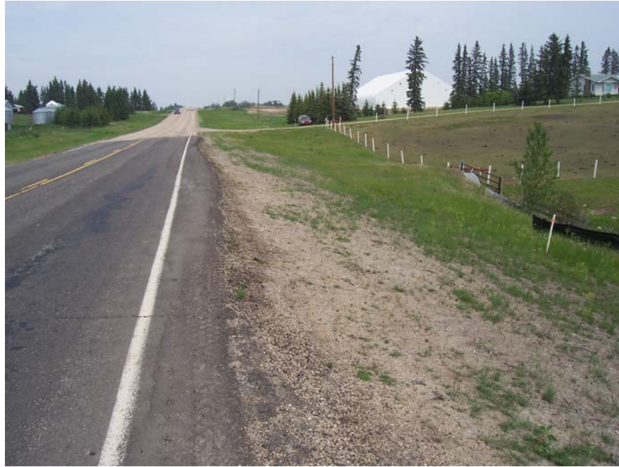
Site general view looking north.
