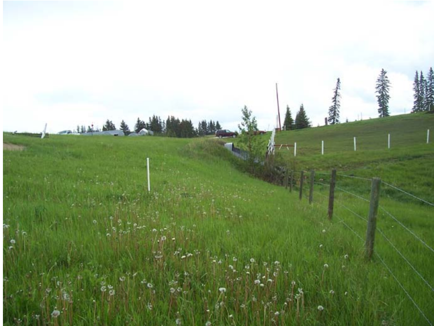
Photo 3 – View of the slide toe roll.
