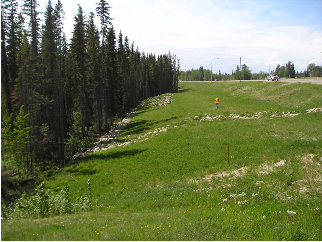
Photo 3 – Berm and toe area (looking west).
