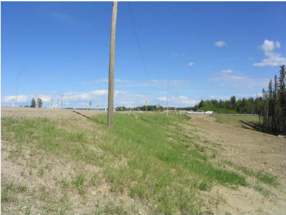
PHOTO 4 LOOKING EAST AT UPPER SLOPE AND TOE BERM
