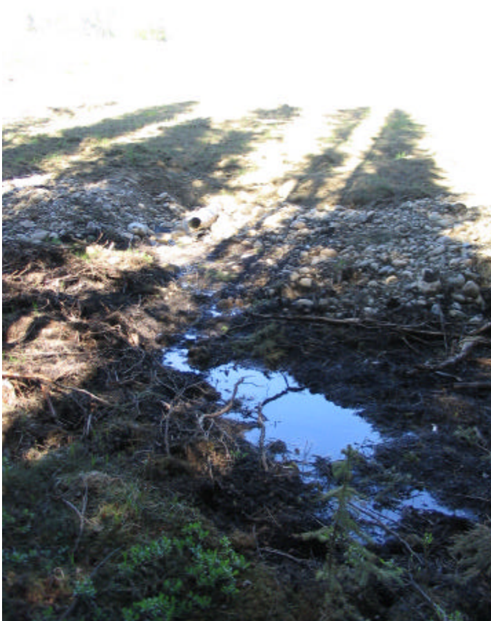
PHOTO 6 OUTFLOW FROM WEST SUBDRAIN OUTLET
