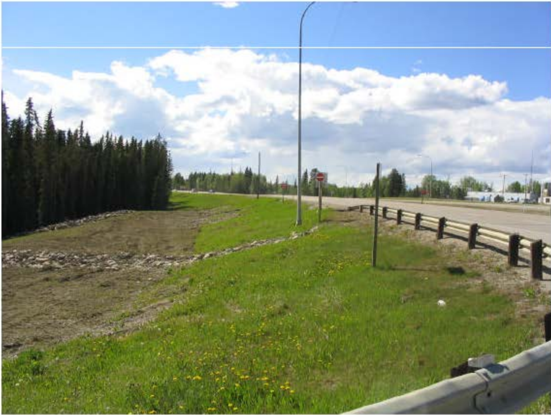
PHOTO 3 LOOKING WEST AT UPPER SLOPE AND TOE BERM
