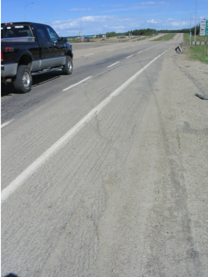
PHOTO 1 AREA OF CRACKS IN PAVEMENT (LOOKING EAST)
