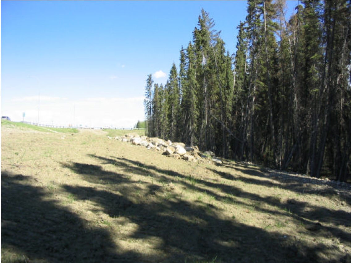
PHOTO 5 LOOKING EAST AT LOWER SLOPE AND RIP RAP FACING
