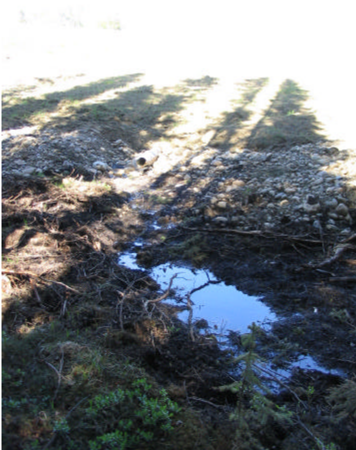
PHOTO 6 OUTFLOW FROM WEST SUBDRAIN OUTLET
