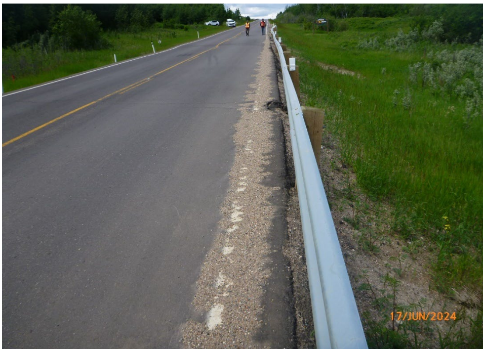
Photo 6 New guardrail posts offset approximately 200 mm from previous location. Photo taken June 17, 2024, facing north.
