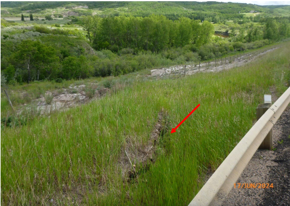
Photo 8 Large ground crack (indicated by red arrow) observed in the east highway embankment slope. Photo taken June 17, 2024, facing east.
