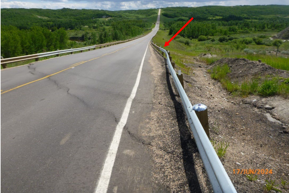
Photo 8 Large ground crack (indicated by red arrow) observed in the east highway embankment slope. Photo taken June 17, 2024, facing east.
