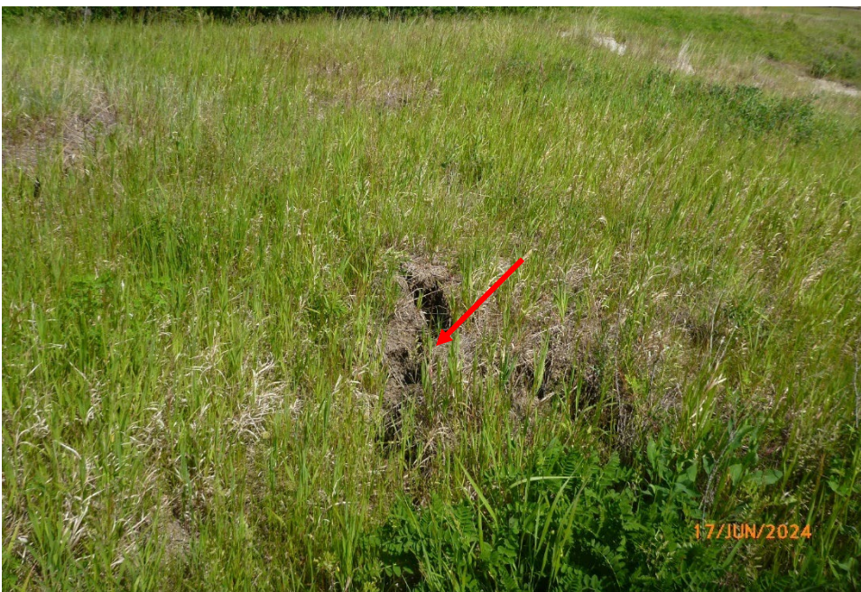
Photo 10 Ground cracking (indicated by red arrow) observed west of the highway embankment. Photo taken June 17, 2024, facing northeast.
