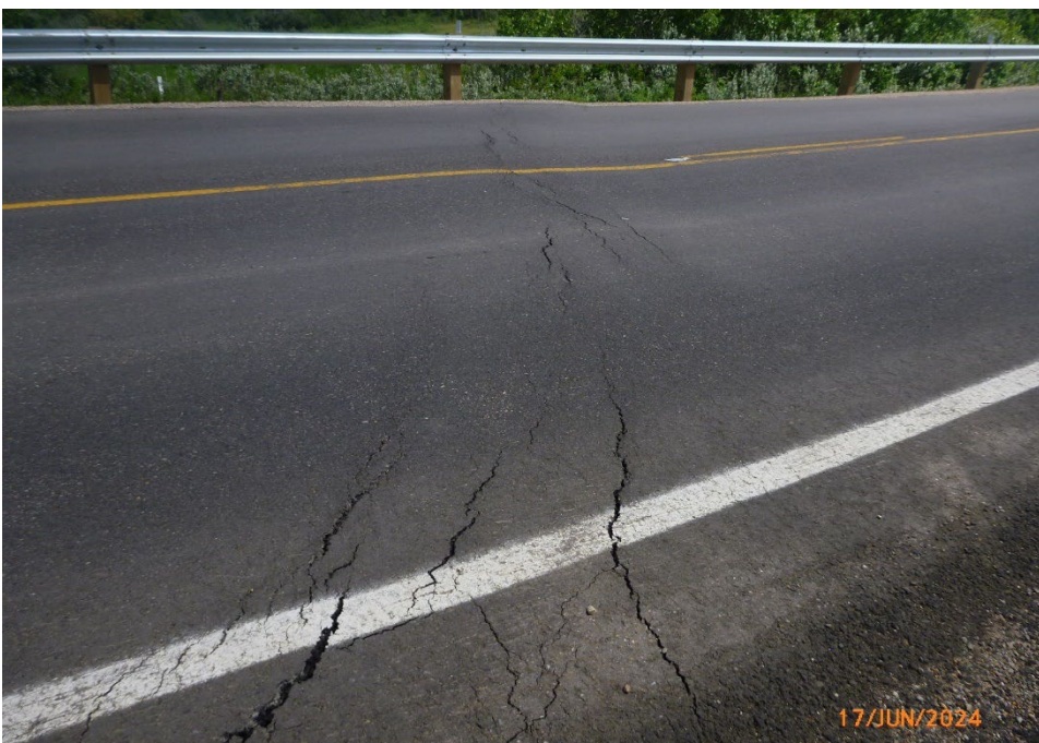
Photo 4 Pavement cracks and settlement observed near the north extent of the site are already showing through a recent pavement patch completed in late-2023 or early-2024. Photo taken June 17, 2024 facing east.
