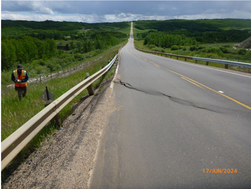
Photo 6 New guardrail posts offset approximately 200 mm from previous location. Photo taken June 17, 2024, facing north.
