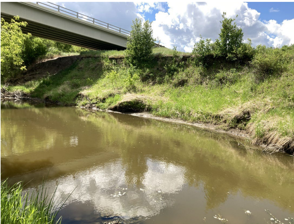
Photo 6 No significant changes to the slide on the south abutment were observed between the 2022 and 2024 inspections. Photo taken June 17, 2024, facing southwest.
