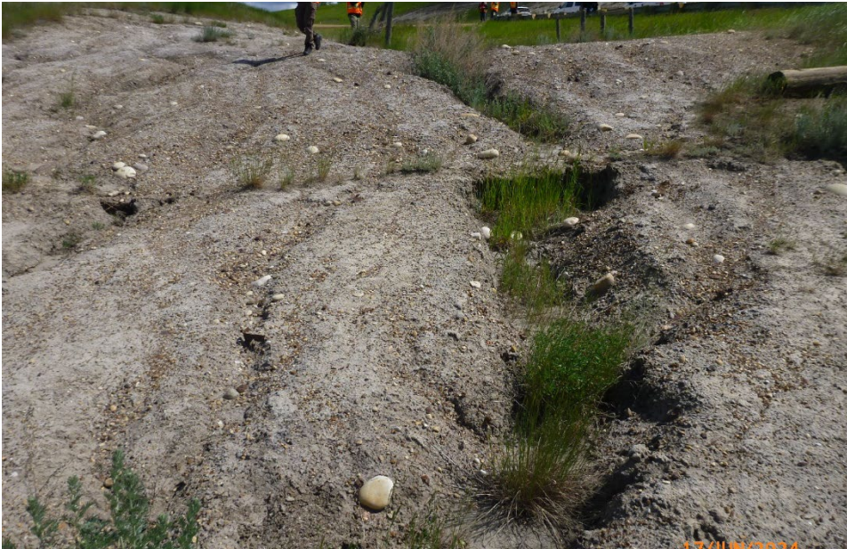
Photo 2 Vegetation and sediment build-up at the catch basin structure at the culvert inlet. Photo taken June 17, 2024, facing northeast.
