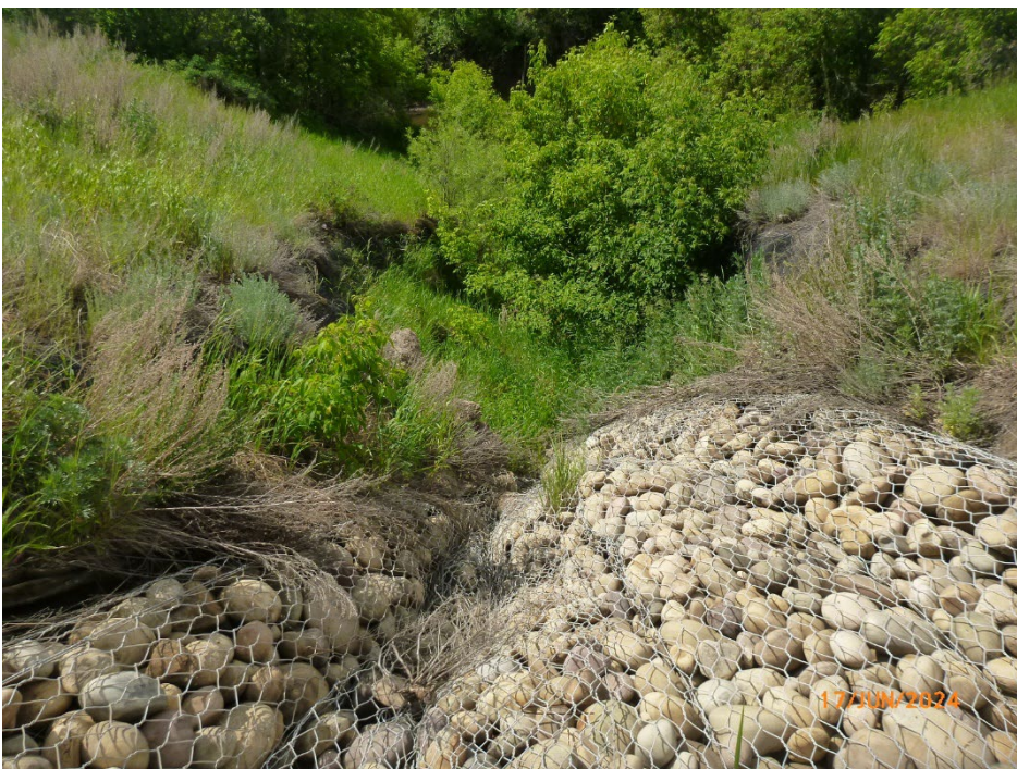
Photo 4 Erosion gully downstream of the failing gabion mattress in the east (northbound) ditch. Dense vegetation (grass, shrubs, and trees) growing within erosion gully. Photo taken June 17, 2024, facing south.
