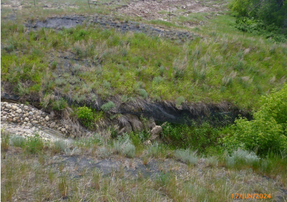
Photo 6 No significant changes to the slide on the south abutment were observed between the 2022 and 2024 inspections. Photo taken June 17, 2024, facing southwest.
