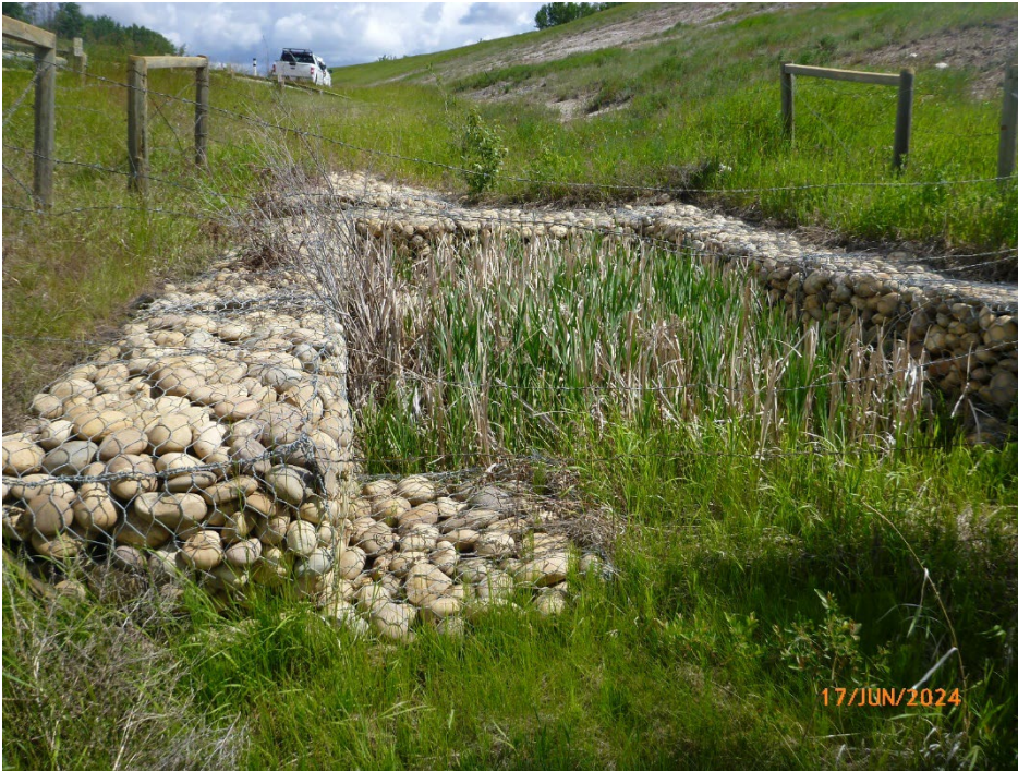
Photo 4 Erosion gully downstream of the failing gabion mattress in the east (northbound) ditch. Dense vegetation (grass, shrubs, and trees) growing within erosion gully. Photo taken June 17, 2024, facing south.
