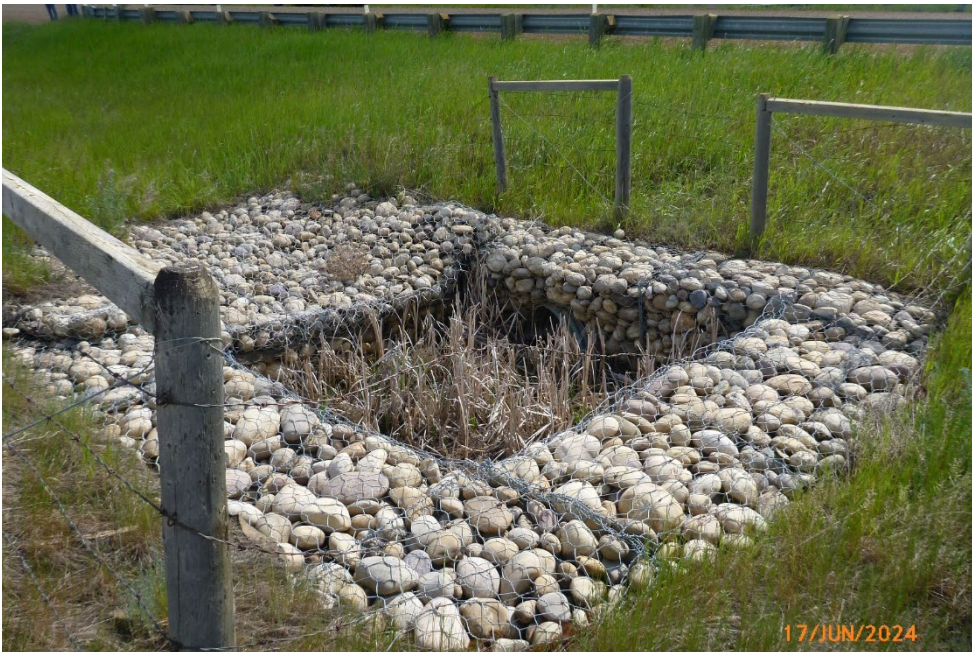
Photo 2 Vegetation and sediment build-up at the catch basin structure at the culvert inlet. Photo taken June 17, 2024, facing northeast.
