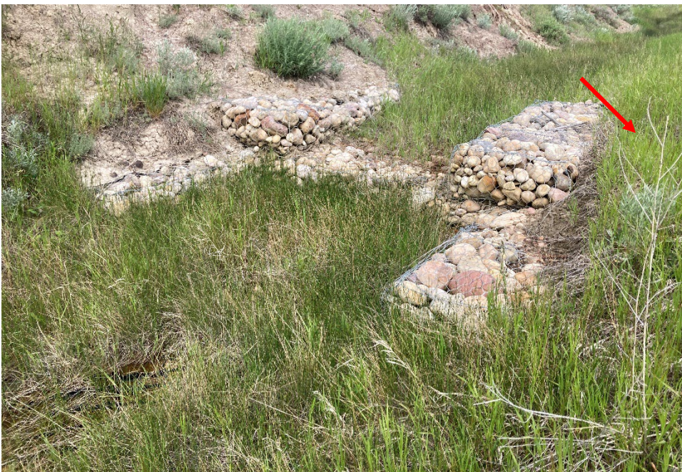
Photo 4 The gabion basket drop structure near the south extent of the site appears to be in good condition. A sinkhole (approximately 0.5 m in diameter and 0.5 m deep, location indicated by red arrow) was observed near the east (left) edge of the drop structure. Photo taken June 18, 2024, facing north.
