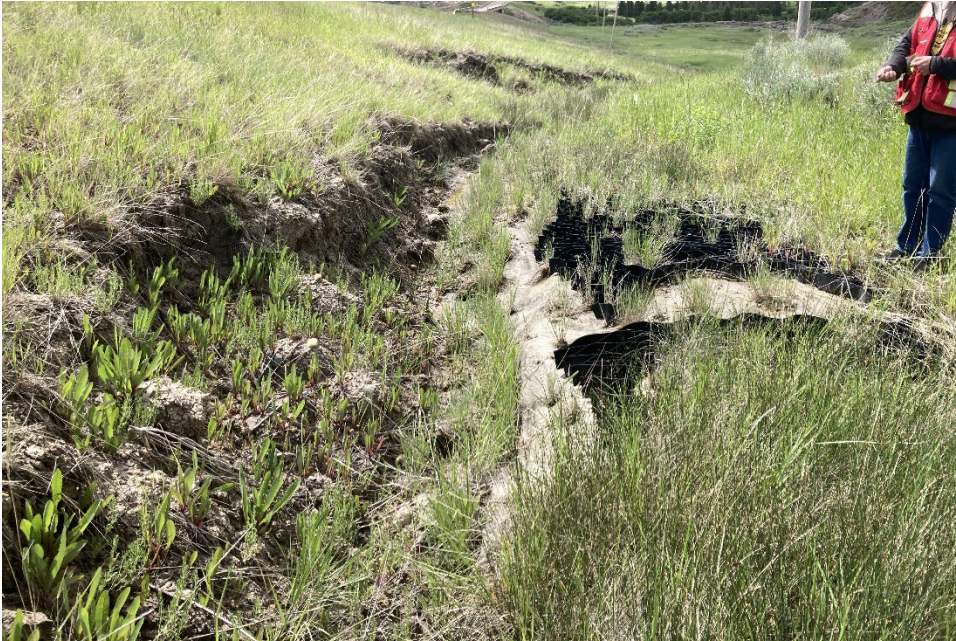
Photo 4 The gabion basket drop structure near the south extent of the site appears to be in good condition. A sinkhole (approximately 0.5 m in diameter and 0.5 m deep, location indicated by red arrow) was observed near the east (left) edge of the drop structure. Photo taken June 18, 2024, facing north.
