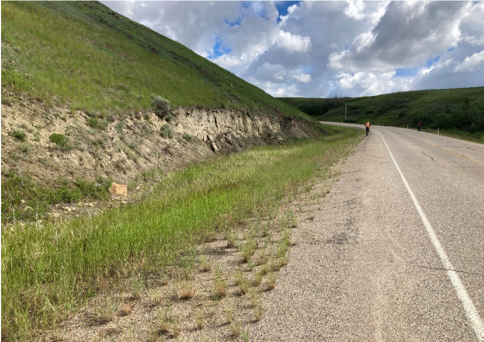
Photo 10 Erosion in the west (southbound) ditch is eroding the highway embankment slope and has reached the edge of the pavement. Photo taken June 18, 2024, facing northeast.
