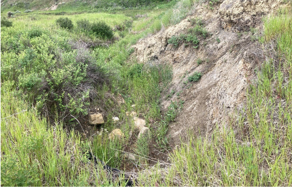
Photo 8 The geocell armouring in the west (southbound) ditch is undermined and a vertical erosion face is approximately 5 m downstream of the gabion basket drop structure. Photo taken June 18, 2024, facing northeast.
