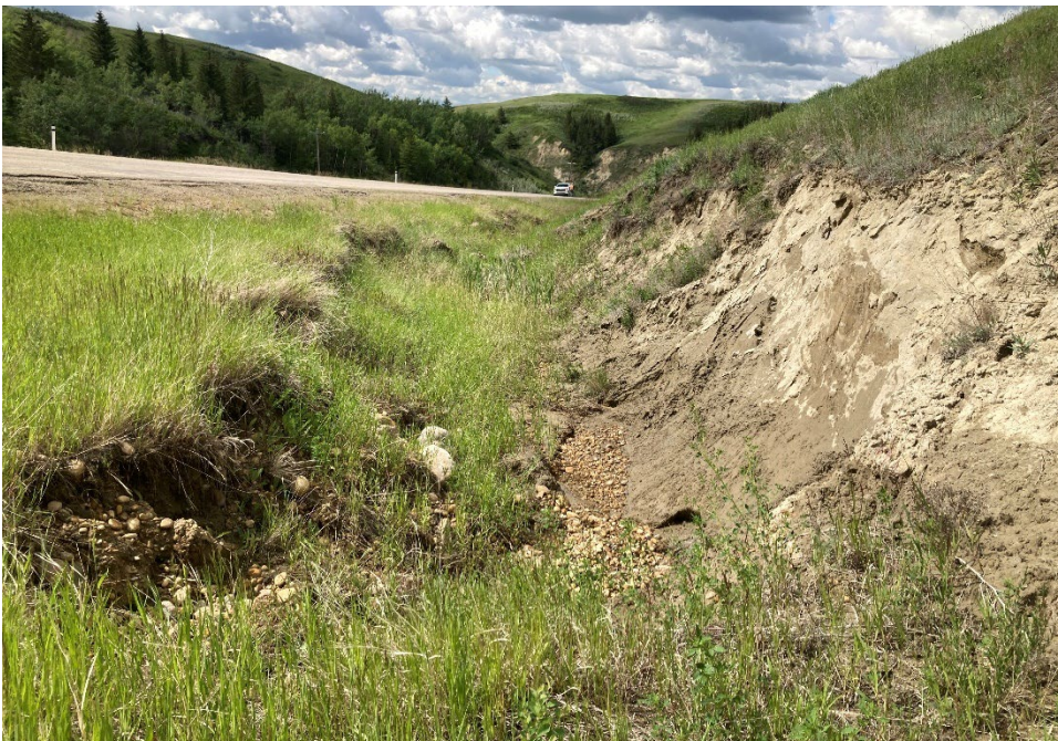
Photo 12 Ditch erosion at the north extent of the site along the toe of the natural slope. Photo taken June 18, 2024, facing southwest.
