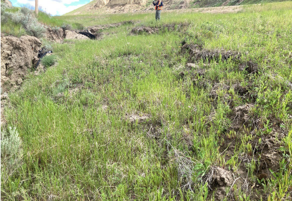
Photo 2 The geocell armoring at the south extent of the site has failed and is being undermined. The degree of erosion appears similar as during the 2023 inspection. Photo taken June 18, 2024, facing north.
