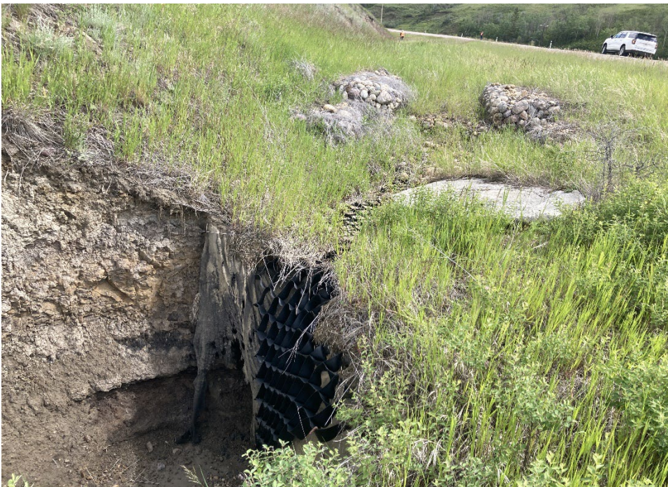
Photo 8 The geocell armouring in the west (southbound) ditch is undermined and a vertical erosion face is approximately 5 m downstream of the gabion basket drop structure. Photo taken June 18, 2024, facing northeast.
