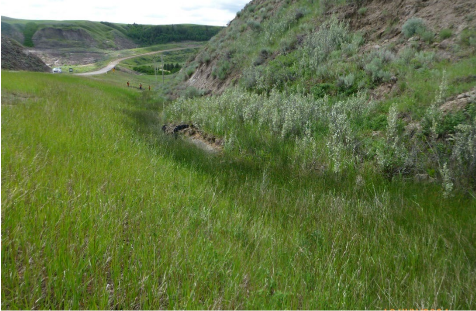
Photo 6 Erosion in the east (northbound) lane ditch near the midpoint of the site appears to have expanded between the 2023 and 2024 inspections and is less than 1 m from the edge of pavement. Photo taken June 18, 2024, facing south.
