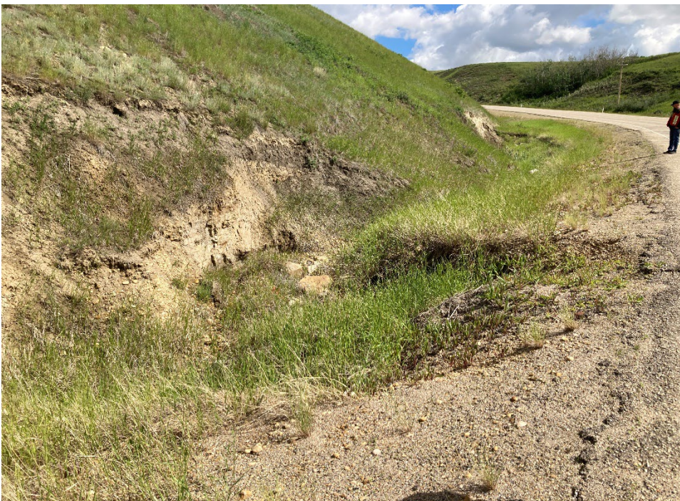
Photo 10 Erosion in the west (southbound) ditch is eroding the highway embankment slope and has reached the edge of the pavement. Photo taken June 18, 2024, facing northeast.
