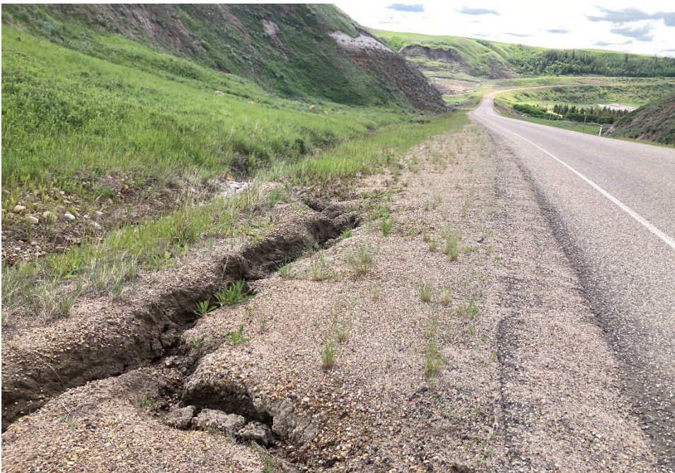
Photo 6 Erosion in the east (northbound) lane ditch near the midpoint of the site appears to have expanded between the 2023 and 2024 inspections and is less than 1 m from the edge of pavement. Photo taken June 18, 2024, facing south.
