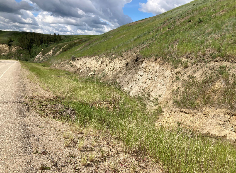
Photo 12 Ditch erosion at the north extent of the site along the toe of the natural slope. Photo taken June 18, 2024, facing southwest.
