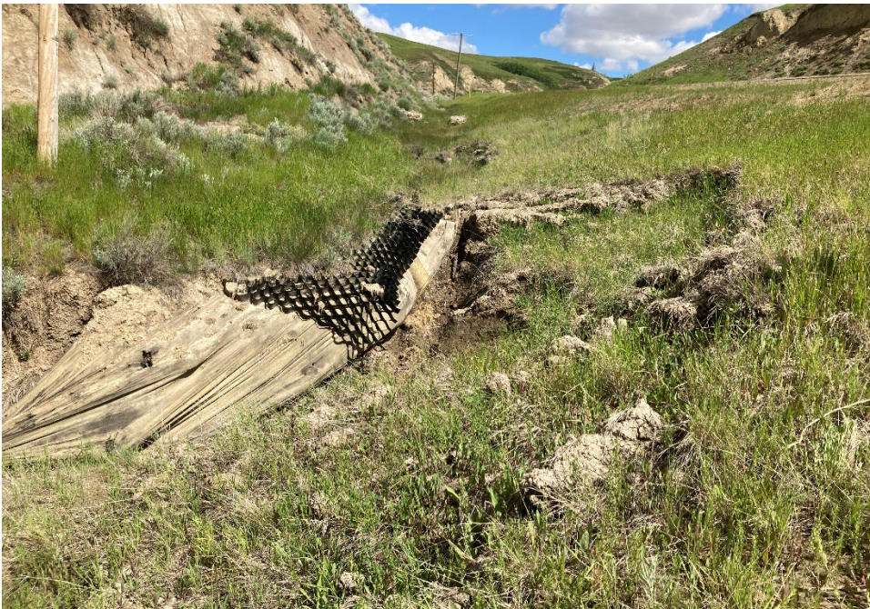
Photo 2 The geocell armoring at the south extent of the site has failed and is being undermined. The degree of erosion appears similar as during the 2023 inspection. Photo taken June 18, 2024, facing north.
