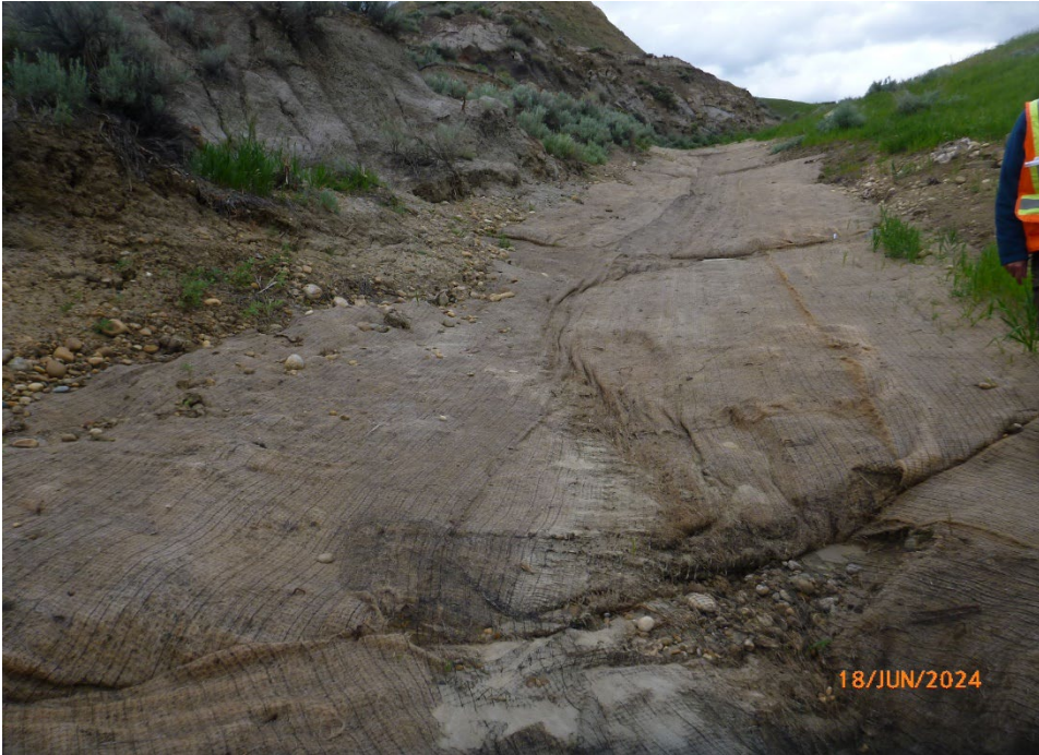
Photo 8 Undermining of the RECP observed in the north ditch near the west extent of the repair. Photo taken June 18, 2024, facing east.
