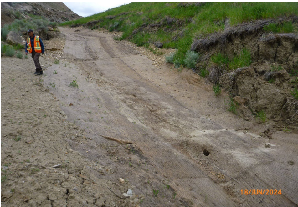
Photo 8 Undermining of the RECP observed in the north ditch near the west extent of the repair. Photo taken June 18, 2024, facing east.
