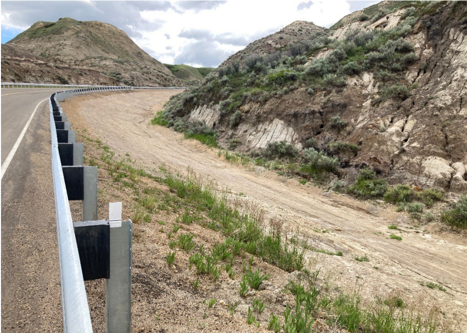
Photo 14 Erosion is ongoing at the outlet of the south ditch repair and is beginning to undermine the RECP. Photo taken June 18, 2024, facing east.
