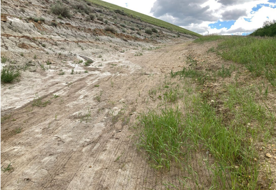
Photo 2 Repair upslope of the ditch block in the north ditch appears to be in good condition and some vegetation growth was observed. Photo taken June 18, 2024, facing west.
