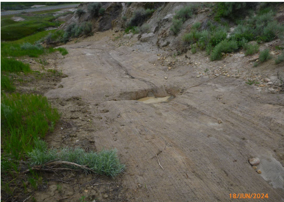
Photo 6 Sinkhole partially filled with water observed in the north ditch, upstream of the steep section at the west extent of the repair, downstream of a draw on the natural slope north of the ditch. Photo taken June 18, 2024, facing west.
