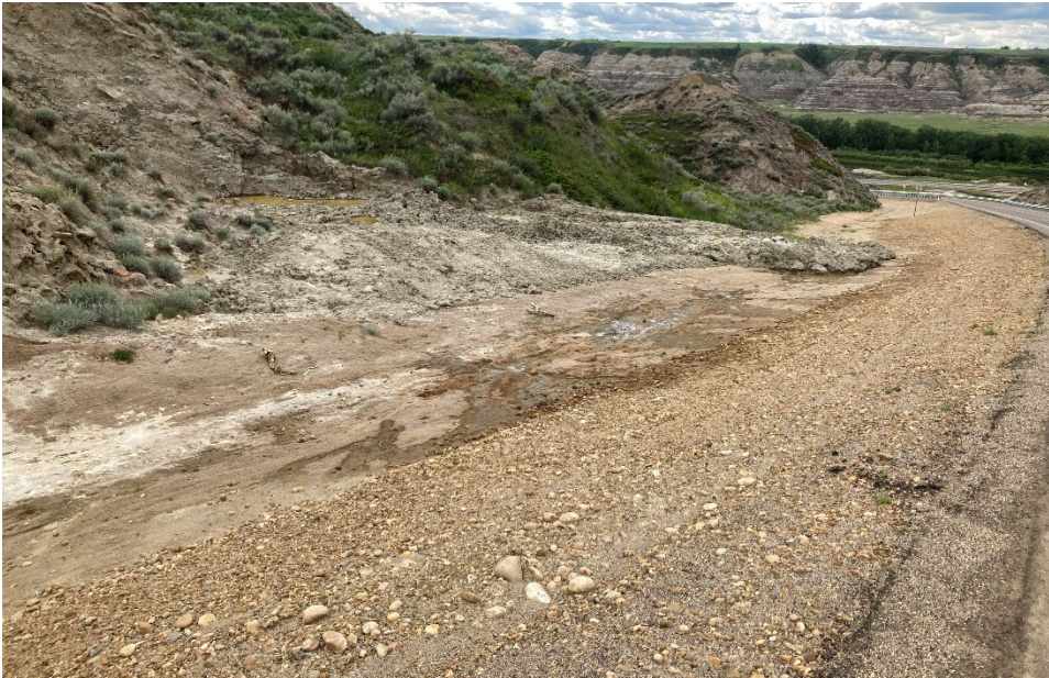
Photo 12 Failed material partially blocking the south ditch. Drainage trench excavated during 2023 construction appears ineffective at conveying seepage from the toe of the slope to the ditch. Photo taken June 18, 2024, facing east.
