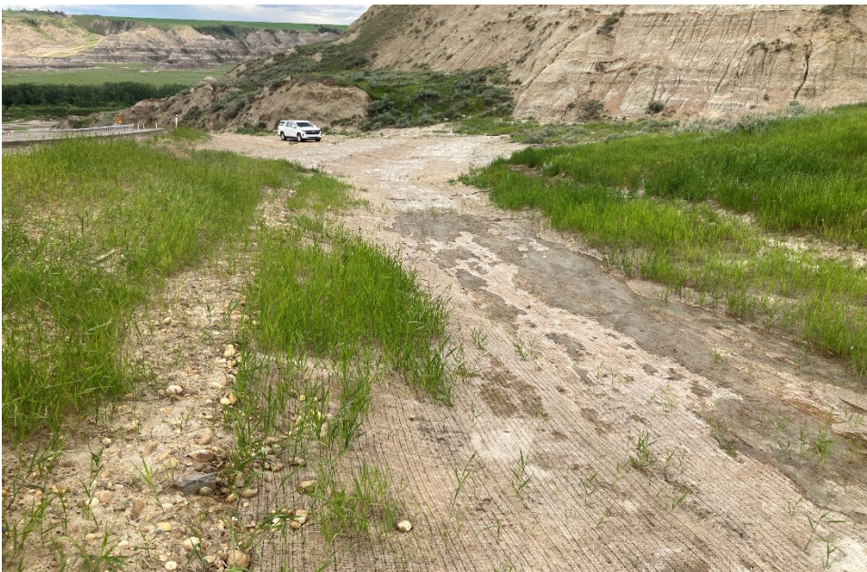
Photo 2 Repair upslope of the ditch block in the north ditch appears to be in good condition and some vegetation growth was observed. Photo taken June 18, 2024, facing west.
