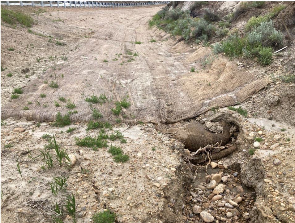
Photo 14 Erosion is ongoing at the outlet of the south ditch repair and is beginning to undermine the RECP. Photo taken June 18, 2024, facing east.
