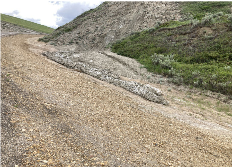
Photo 12 Failed material partially blocking the south ditch. Drainage trench excavated during 2023 construction appears ineffective at conveying seepage from the toe of the slope to the ditch. Photo taken June 18, 2024, facing east.
