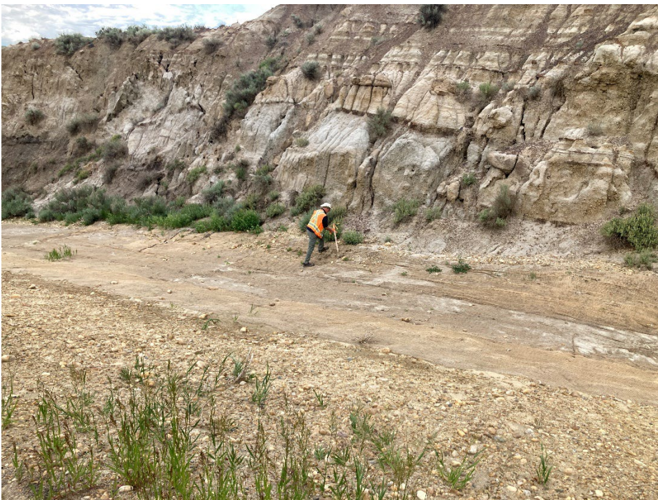
Photo 4 KCB installing a wooden stake to indicate the location of an observed sinkhole on the north ditch side slope. Photo taken June 18, 2024, facing north.
