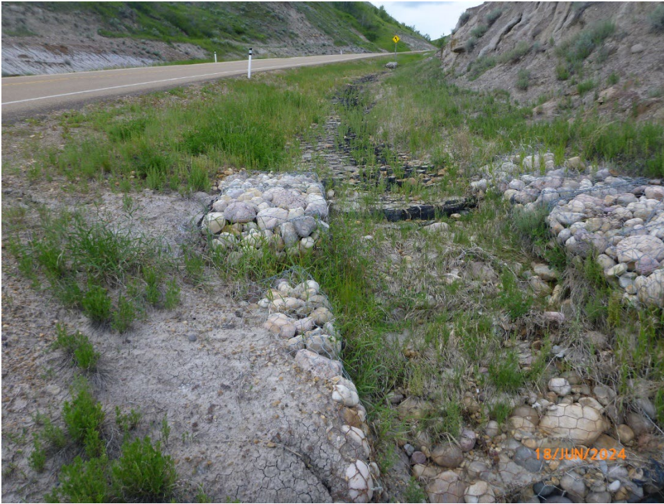
Photo 2 Fine-grained material (silt and clay) has been deposited in the geocell armouring. Photo taken June 18, 2024, facing northwest.
