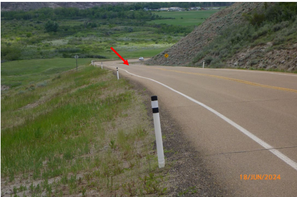
Photo 8 Depressions were observed in the highway surface downhill (southeast, location indicated by red arrow) of the C011 site. Photo taken June 18, 2024, facing southeast.
