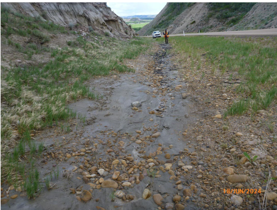
Photo 2 Fine-grained material (silt and clay) has been deposited in the geocell armouring. Photo taken June 18, 2024, facing northwest.
