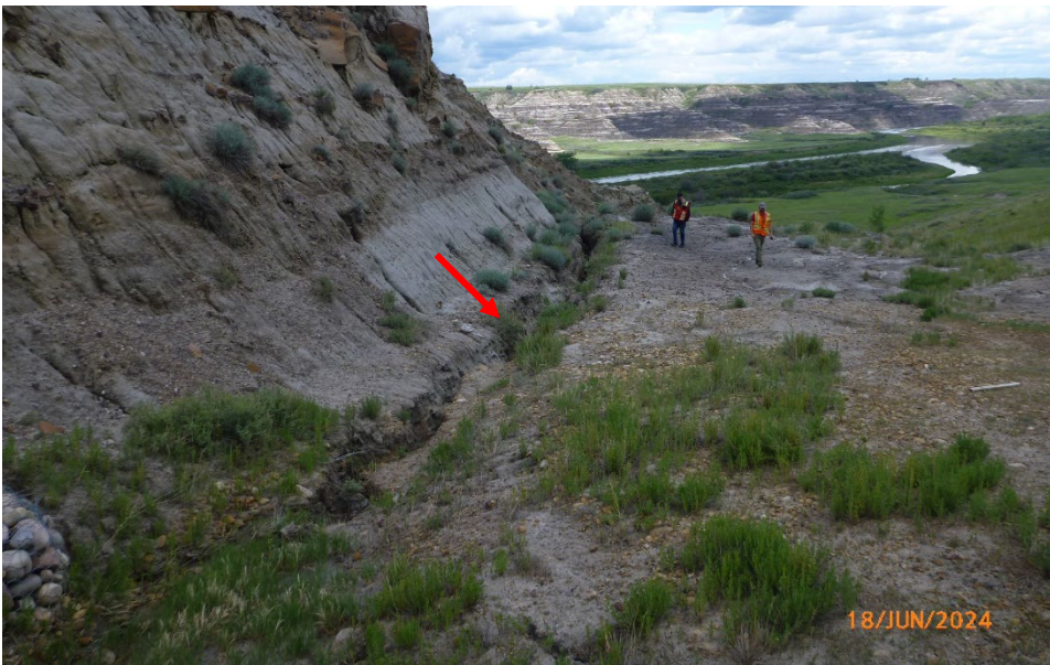
Photo 4 The erosion downstream of the geocell repair and gabions is significantly wider and deeper than during the 2022 inspection (indicated by red arrow). Photo taken June 18, 2024, facing east.
