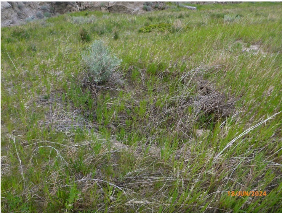
Photo 6 Sinkhole on the highway embankment slope (location shown in Photo 5) appears similar as during the 2022 inspection (approximately 2 m to 3 m in diameter). Photo taken June 19, 2024, facing north.
