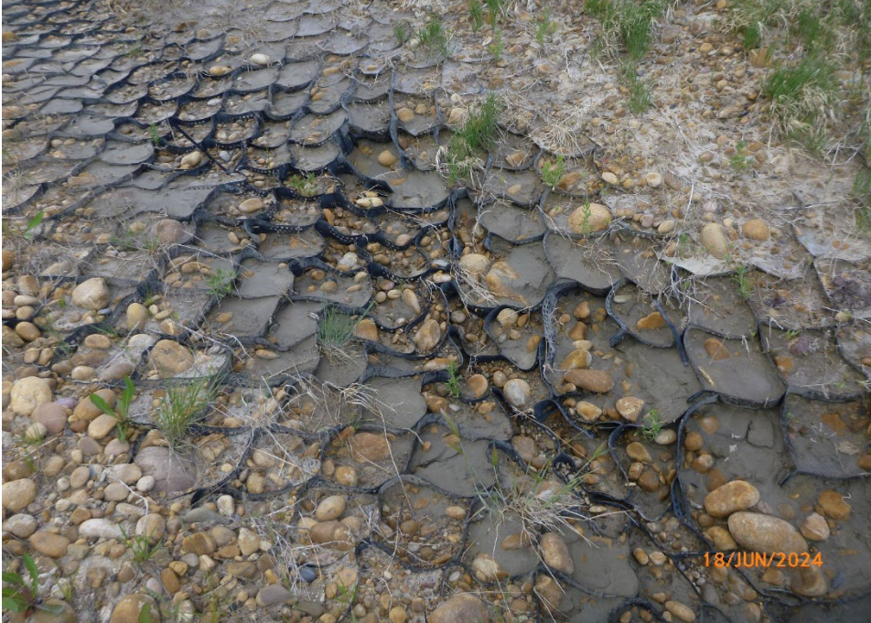
Photo 4 The erosion downstream of the geocell repair and gabions is significantly wider and deeper than during the 2022 inspection (indicated by red arrow). Photo taken June 18, 2024, facing east.
