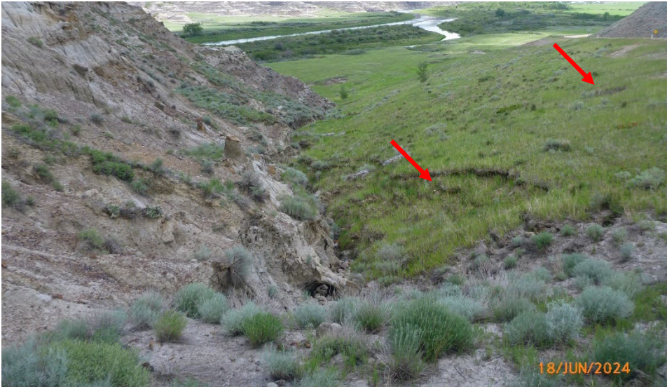
Photo 6 Sinkhole on the highway embankment slope (location shown in Photo 5) appears similar as during the 2022 inspection (approximately 2 m to 3 m in diameter). Photo taken June 19, 2024, facing north.
